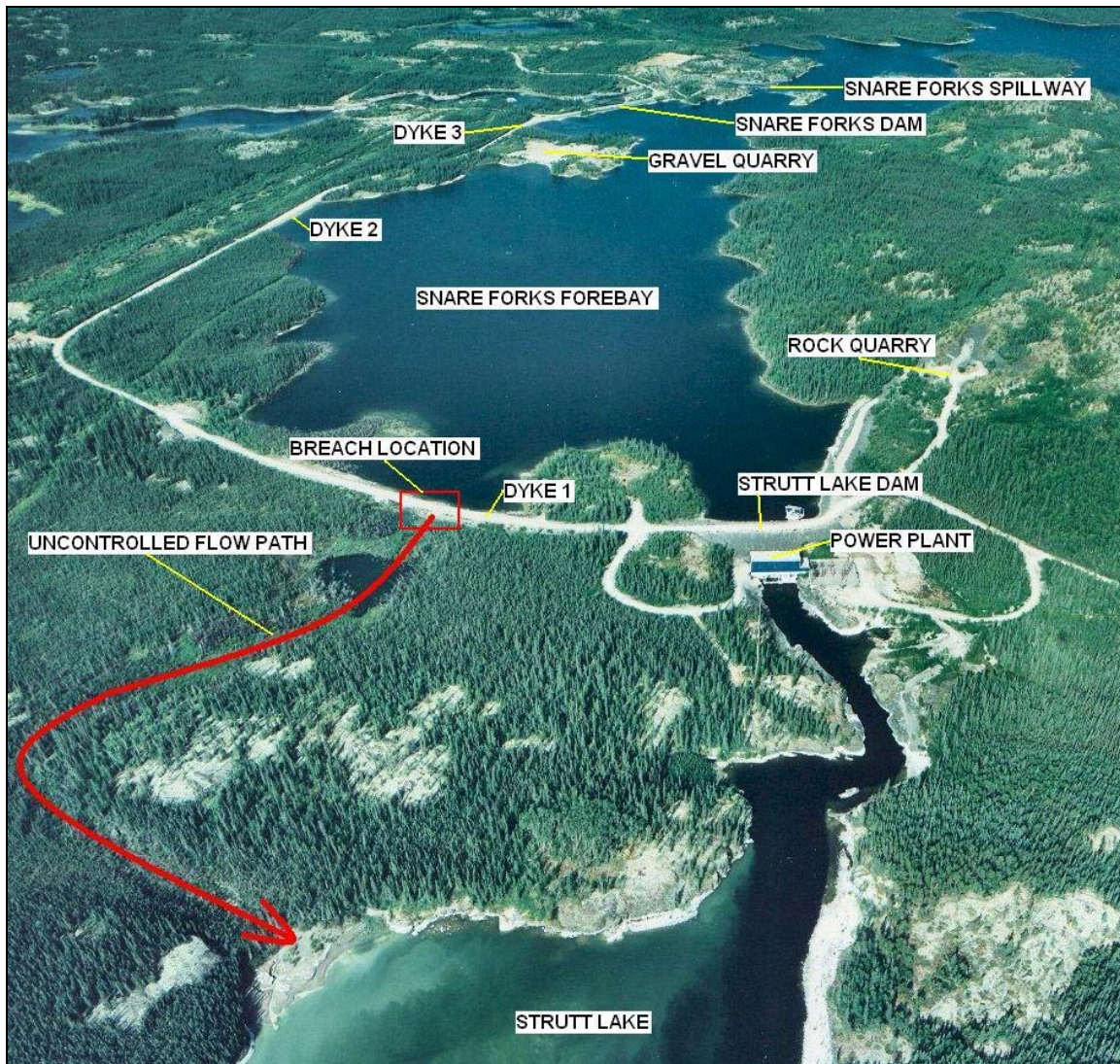
Figure 3: Dyke 1 Breach Discharge Route
