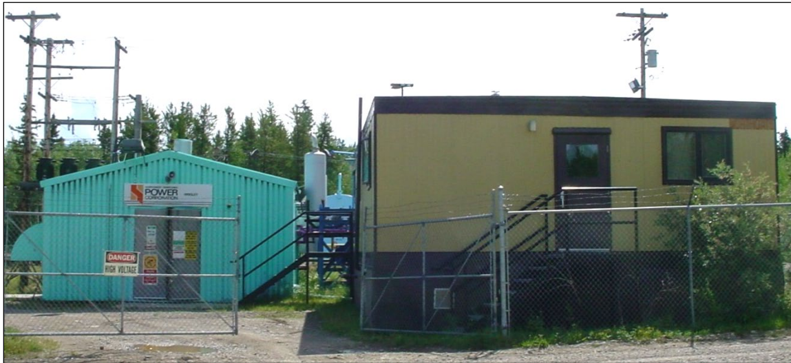
Figure 2: Wrigley Plant – View from North
