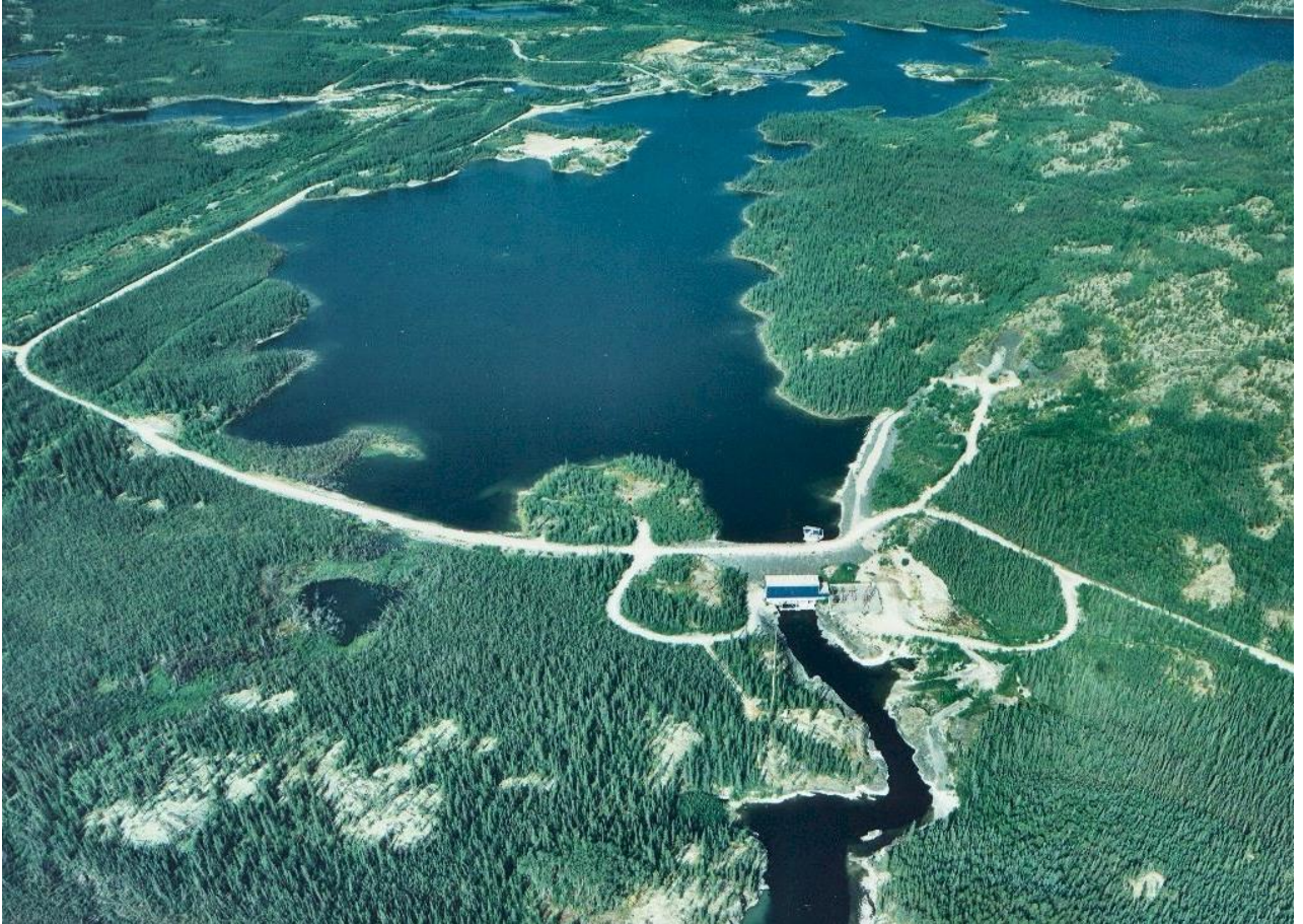
Figure 10: Snare Forks Facility
