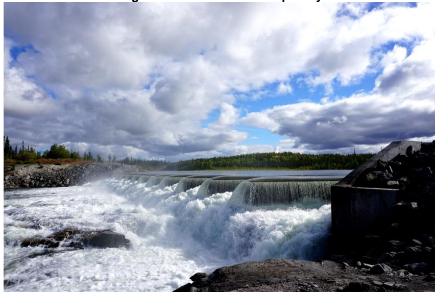
Figure 9: Snare Cascades Spillway
