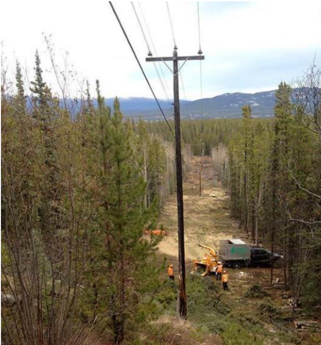
Example of vegetation removal and chipping along powerline ROW ( http://yukontreeservices.ca/photo-gallery/chipping-hydro-line-right-of-way-mt-mac-whitehorse-yl/ ).
