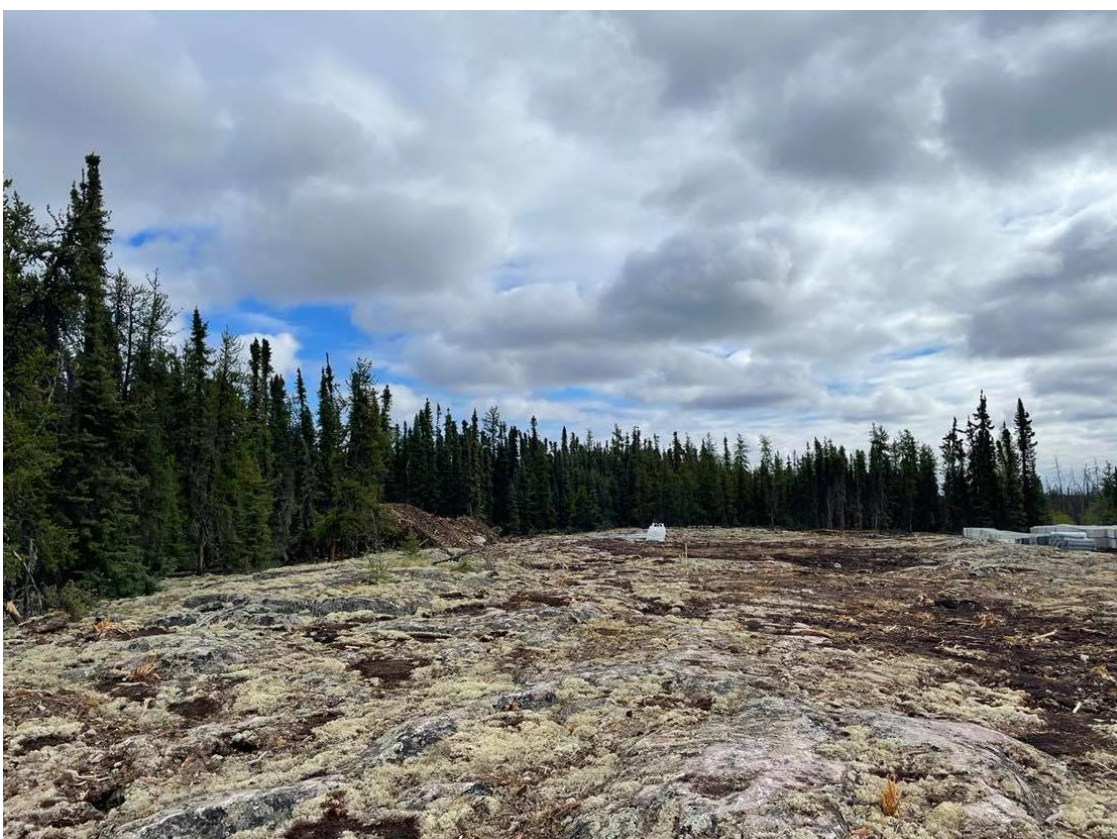
Example of Proper Vegetation Removal with minimal removal of overburden, clean vegetation perimeter with no debris and overburden stockpiled for reclamation once scope of work is completed.
