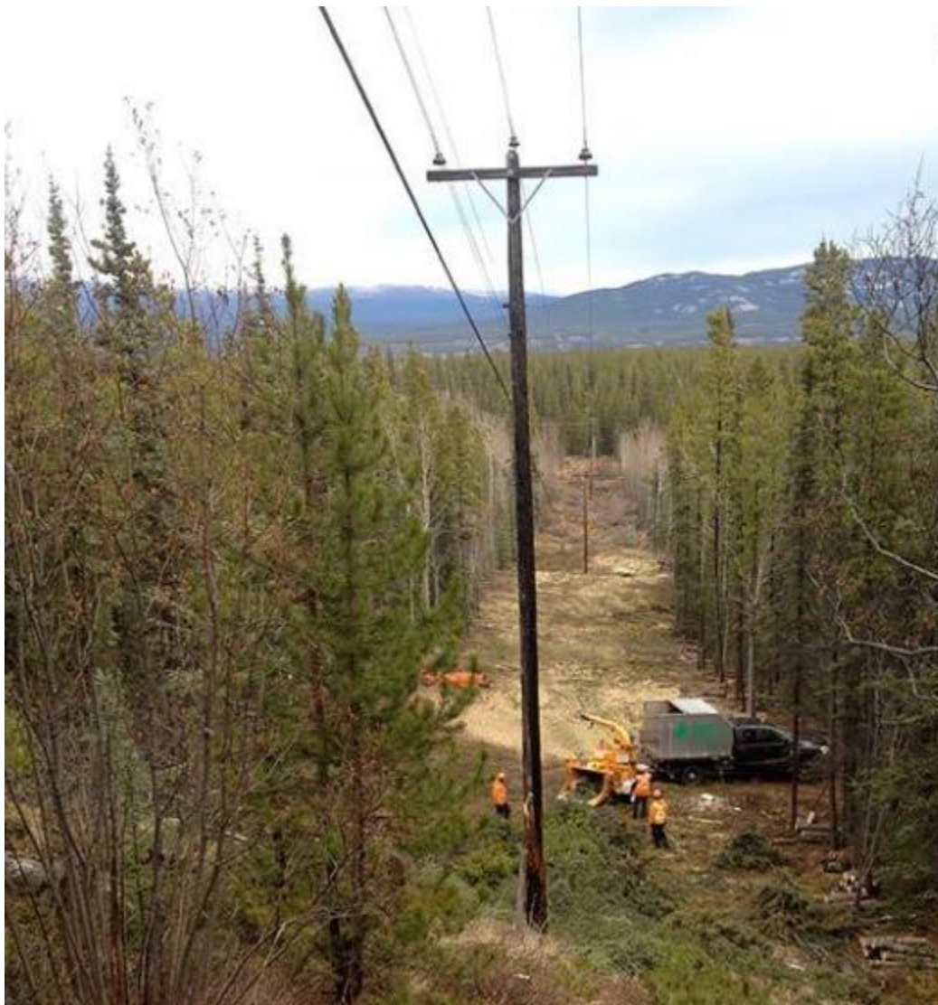
Example of vegetation removal and chipping along powerline ROW ( http://yukontreeservices.ca/photo-gallery/chipping-hydro-line-right-of-way-mt-mac-whitehorse-yt/ ).
