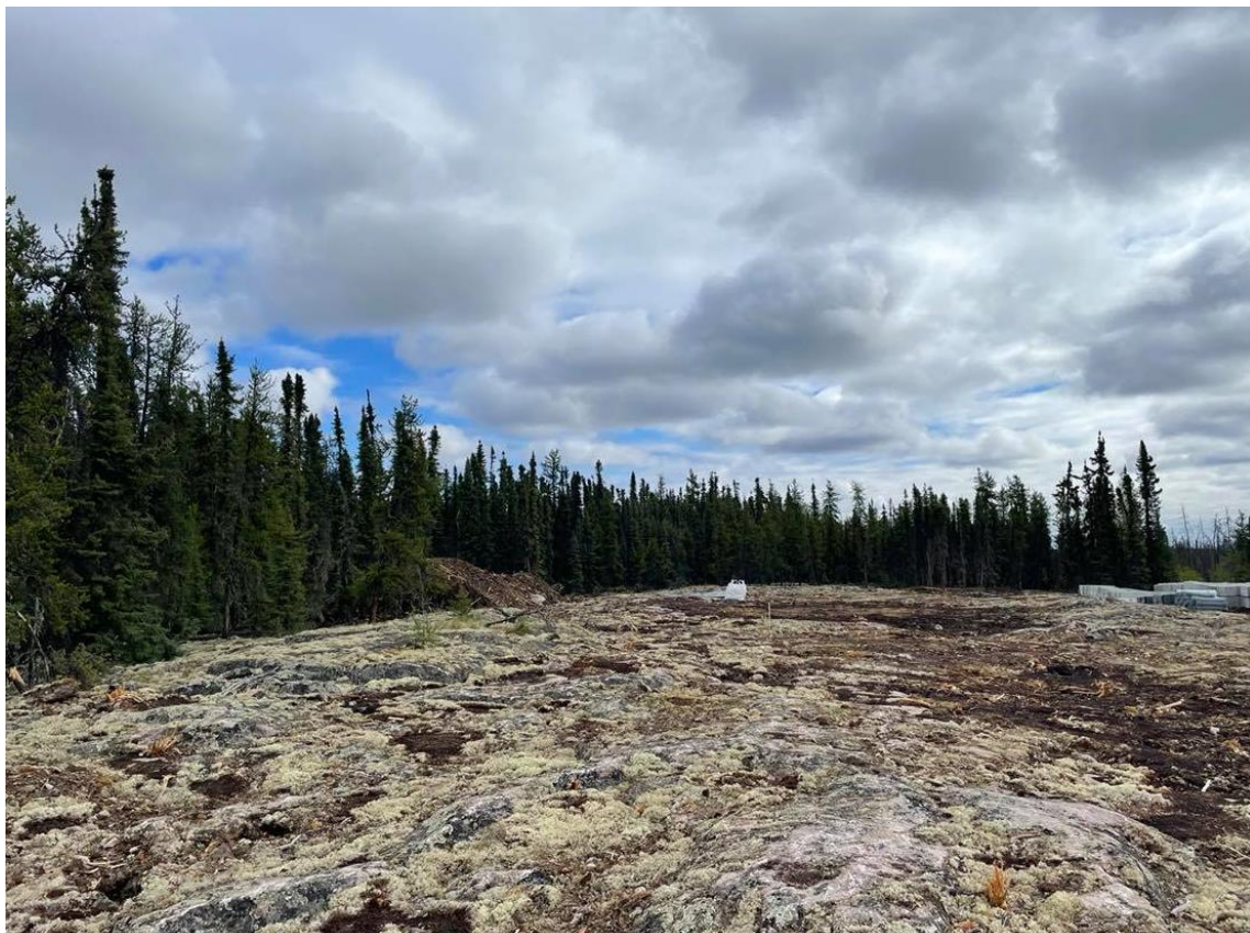
Example of Proper Vegetation Removal with minimal removal of overburden, clean vegetation perimeter with no debris and overburden stockpiled for reclamation once scope of work is completed.
