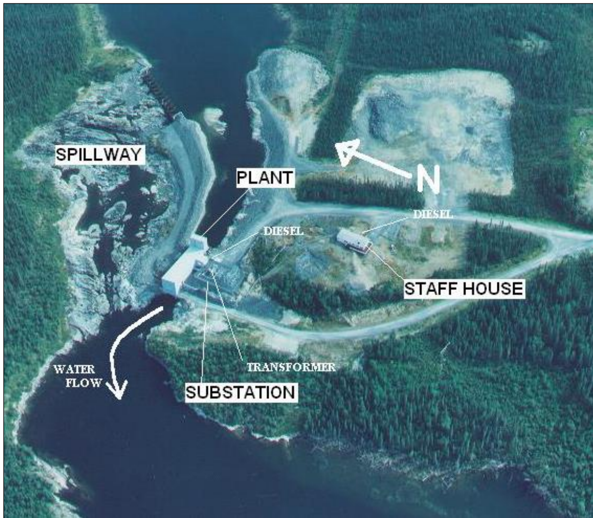
Figure 2-6: Snare Cascades Hydroelectric Facility
