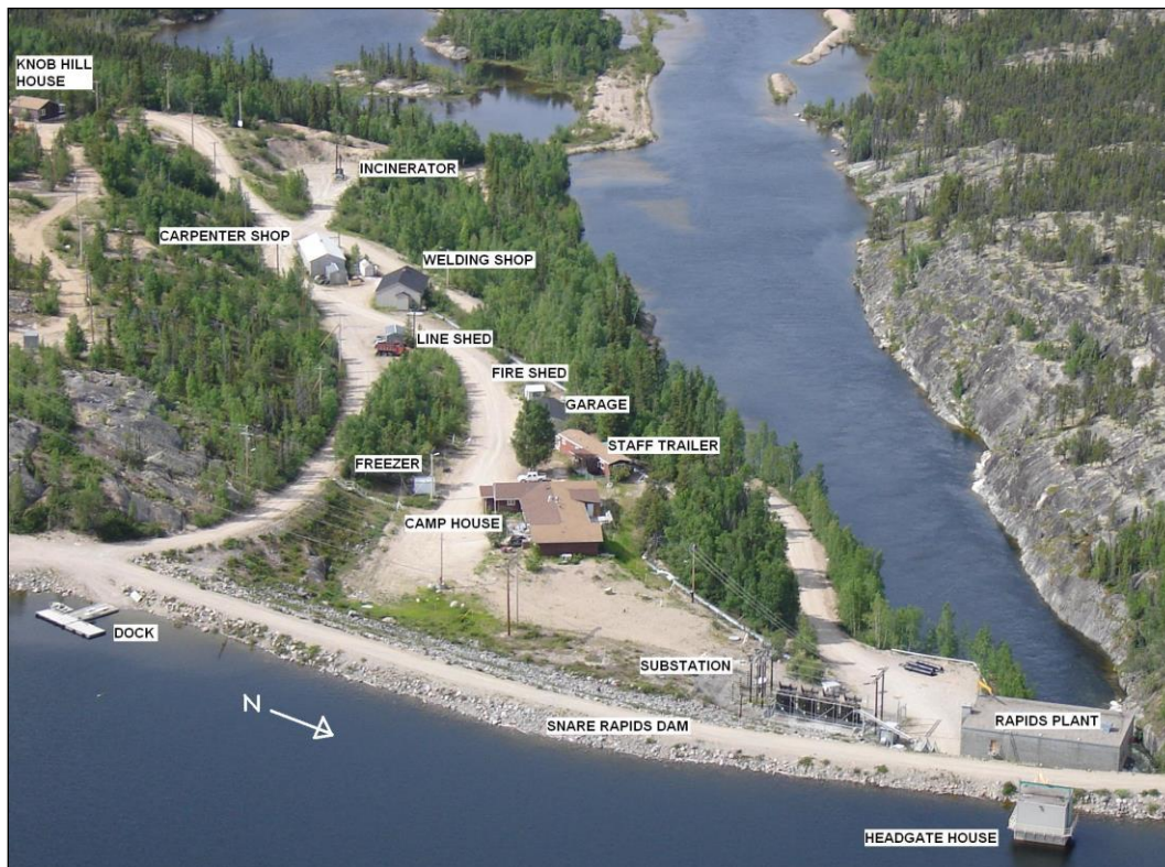
Figure 2-4: Snare Rapids Hydroelectric Facility
