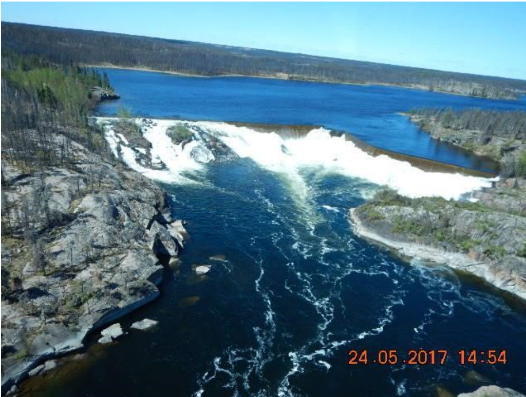
Figure D.33: Taltson Main Spillway
