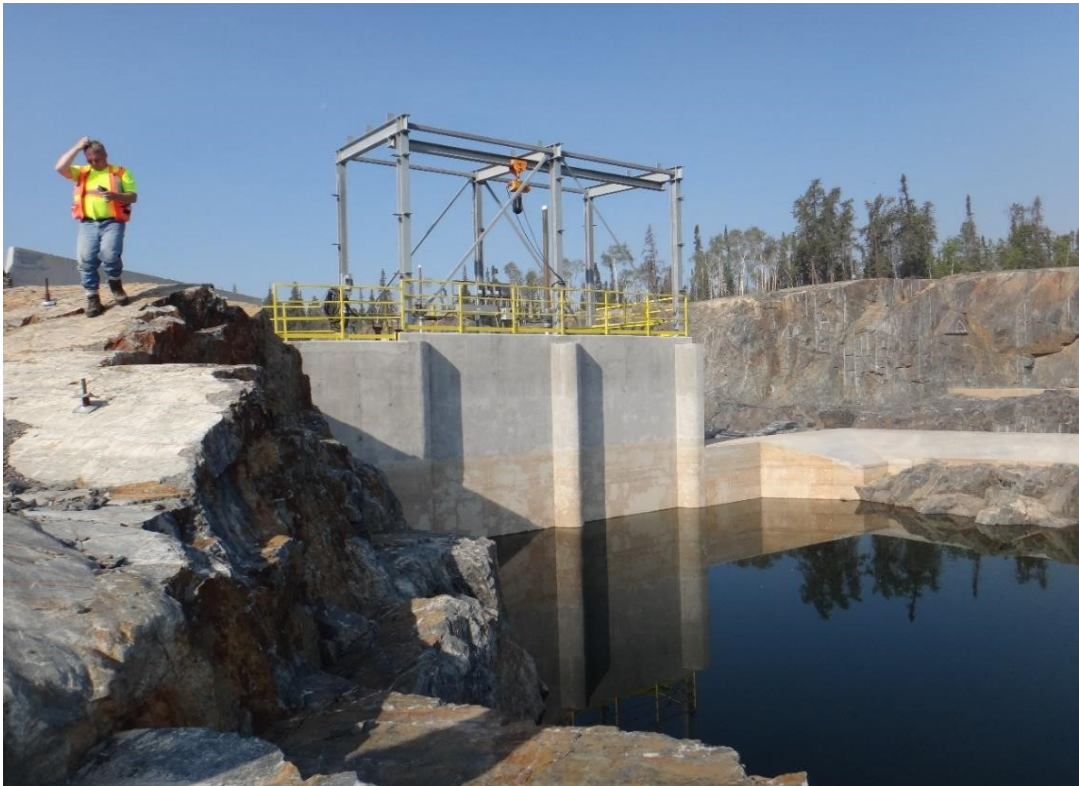
Figure D.42: Bluefish bottom outlet structure
