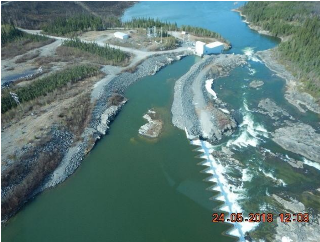
Figure D.15: Snare Cascades Spillway & Power Canal
