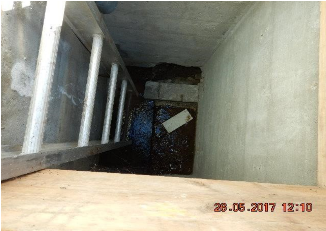
Figure D.3: Snare Rapids Main Dam seepage monitoring weir behind powerhouse
