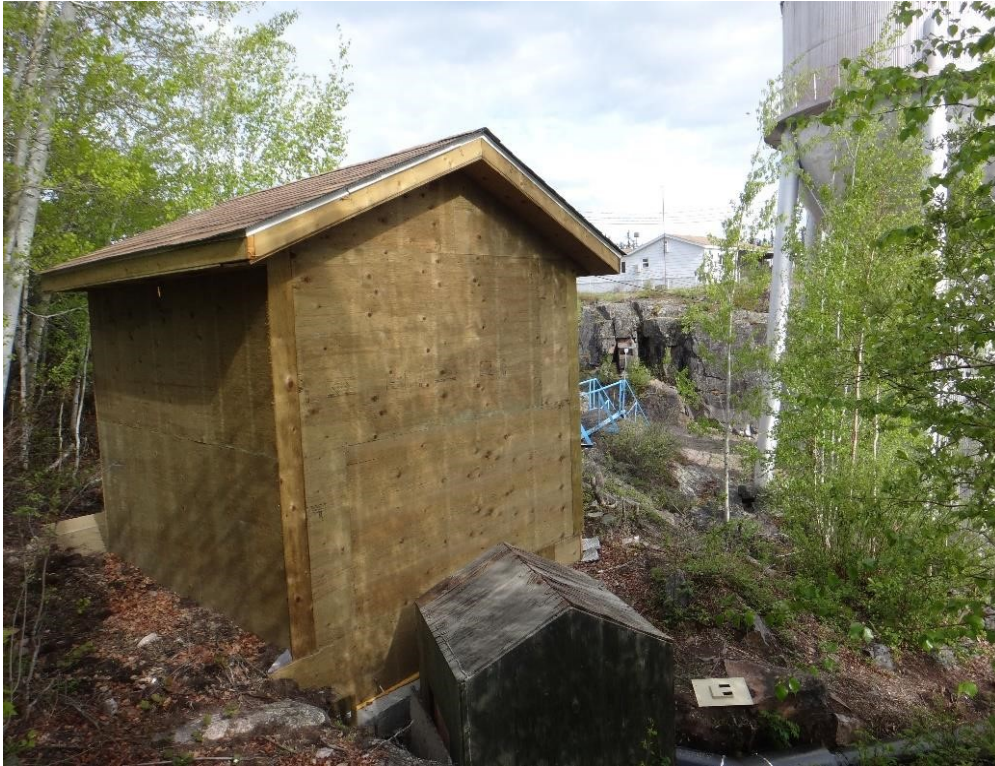
Figure D.37: Taltson Main Dam RB seepage monitoring heated shack
