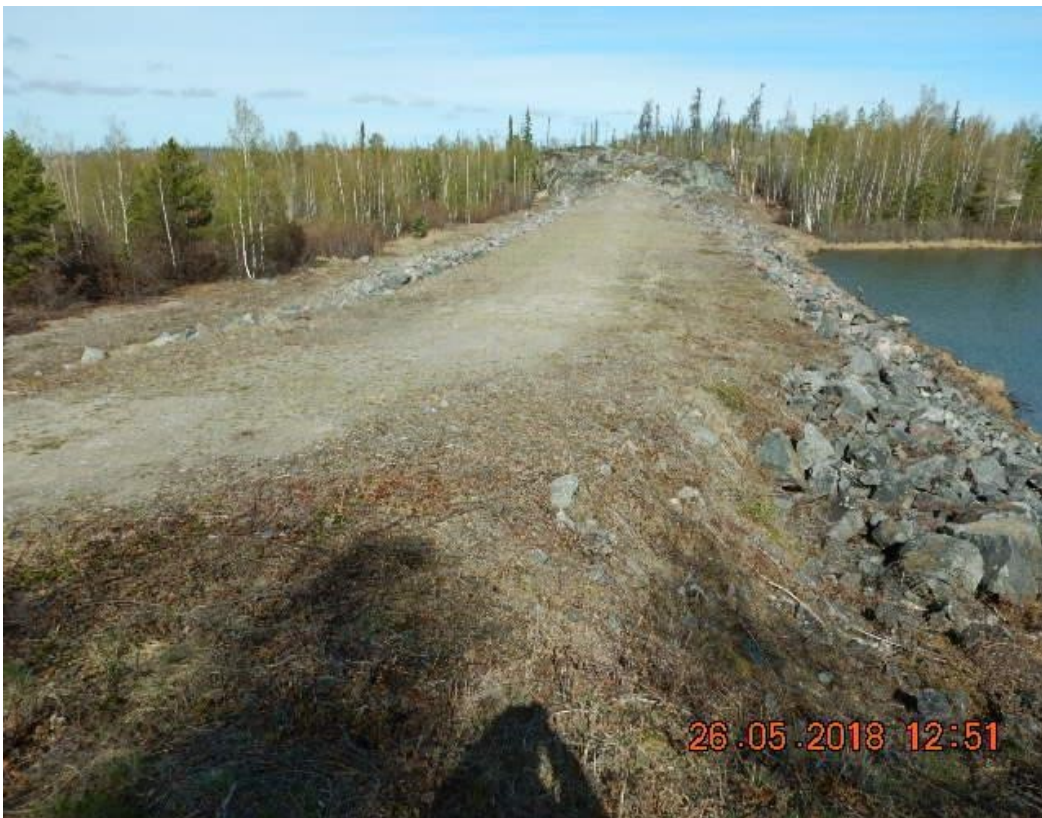
Figure D.12: Snare Falls Side Dam # 1
