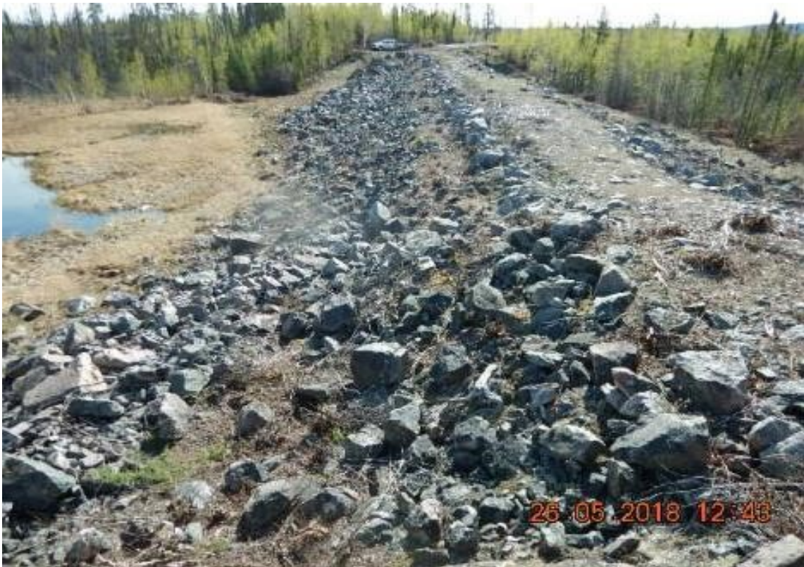
Figure D.14: Snare Falls Side Dam # 2 Upstream
