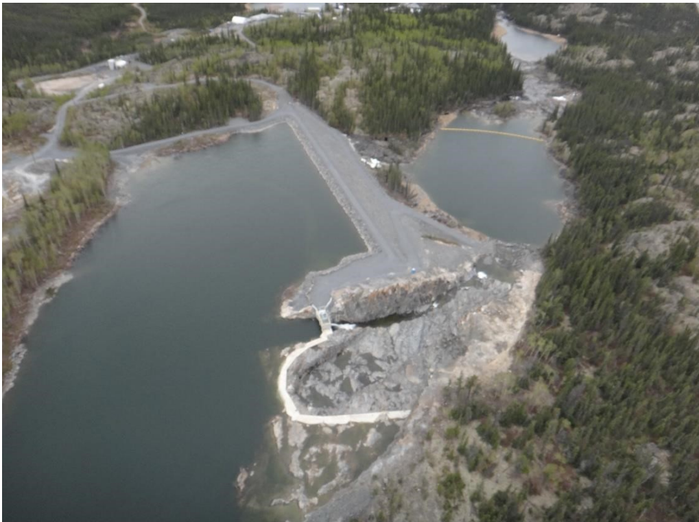
Figure D.40: Bluefish Dam aerial view
