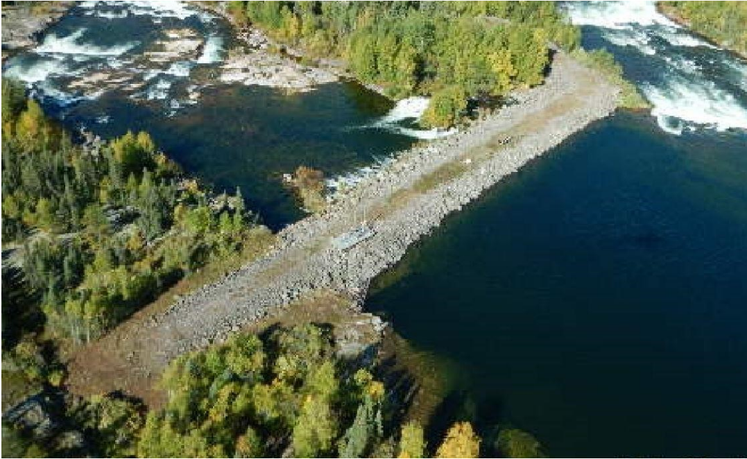
Figure D.27: Nonacho Dam aerial view
