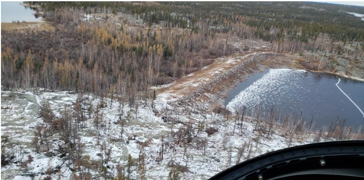
Figure D.8: Snare 4B Dam
