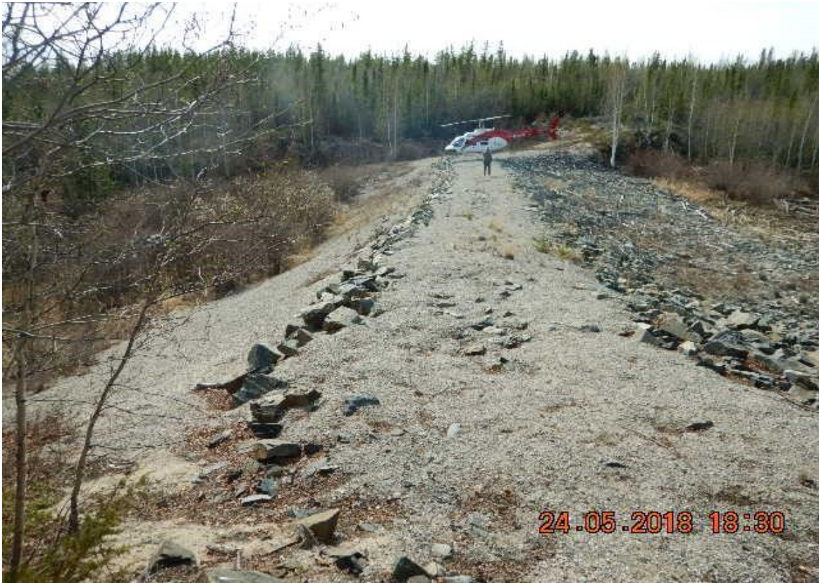
Figure D.9: Snare 9B Dam
