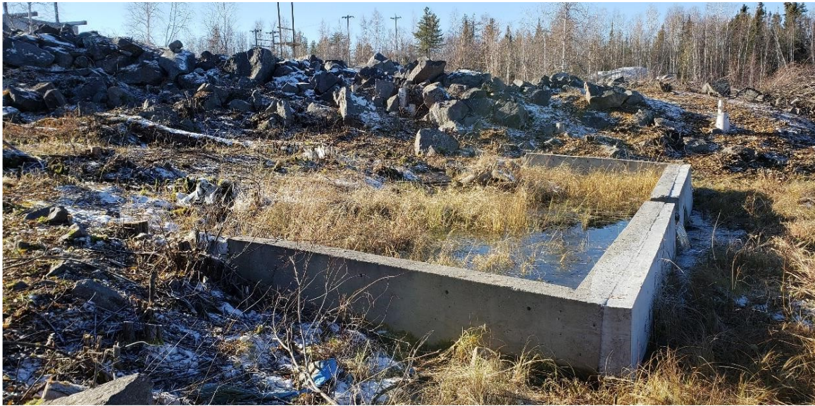
Figure D.7: Snare 5B seepage monitoring weir
