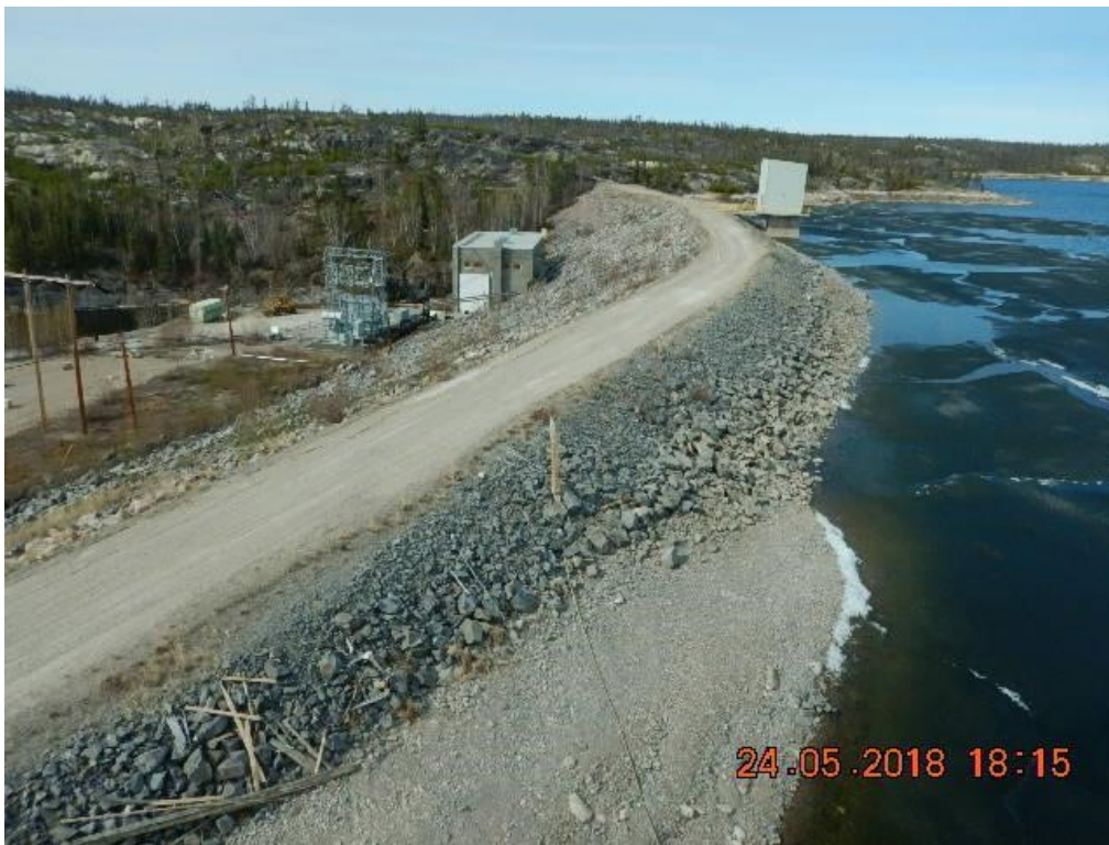
Figure D.2: Snare Rapids Main Dam Upstream
