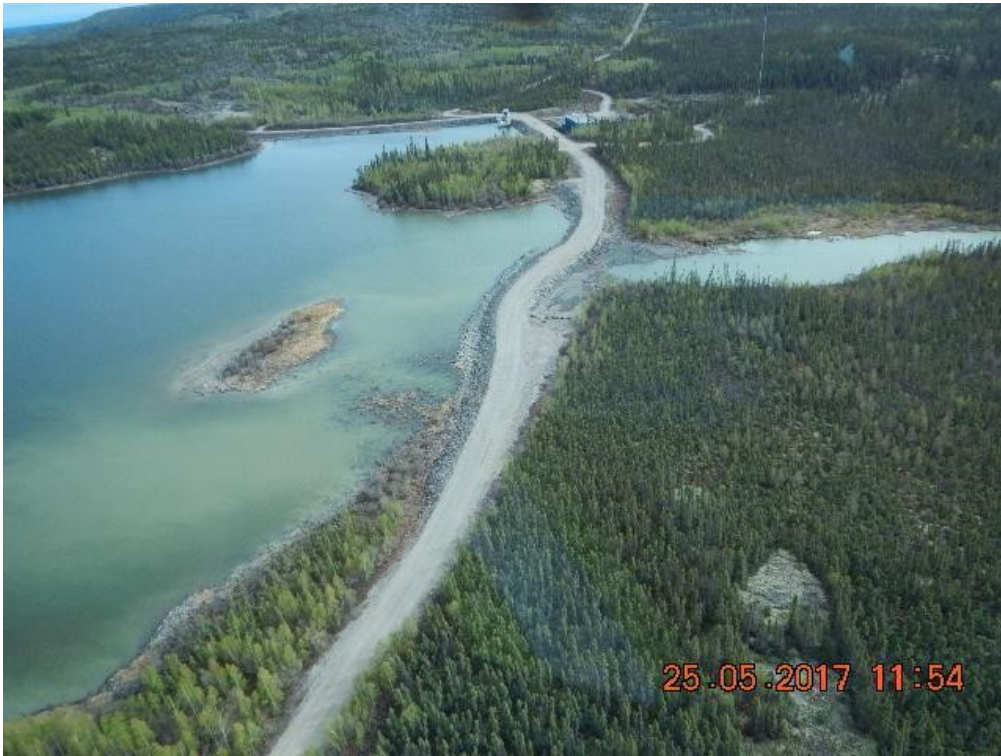
Figure D.17: Snare Forks Dyke 1
