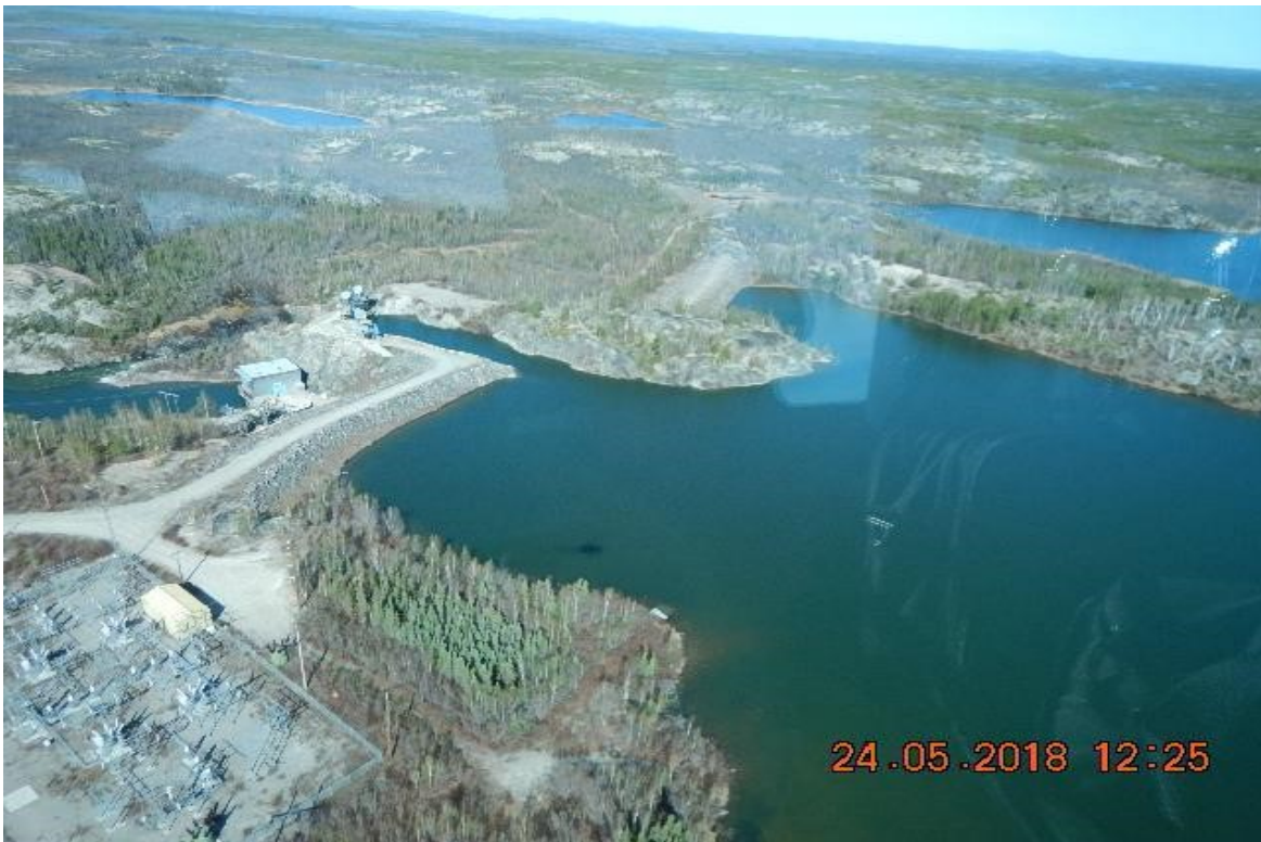
Figure D.10: Snare Falls Main Dam
