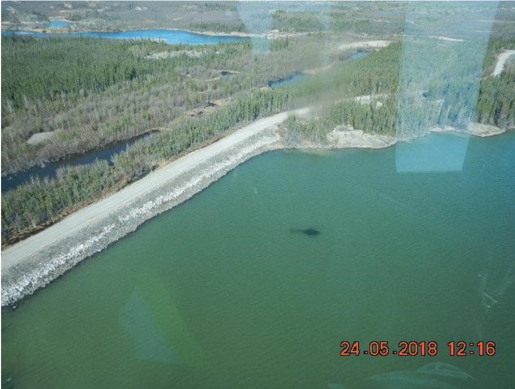
Figure D.19: Snare Forks Dyke 2
