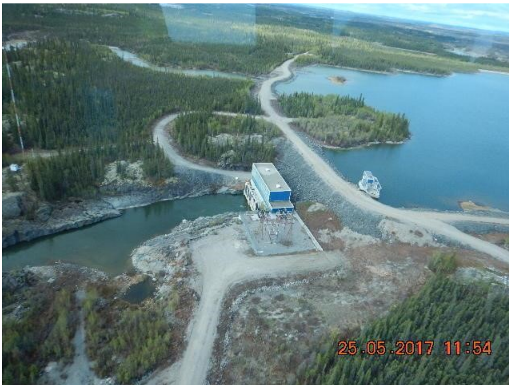
Figure D.16: Snare Forks Strutt Dam & Powerhouse
