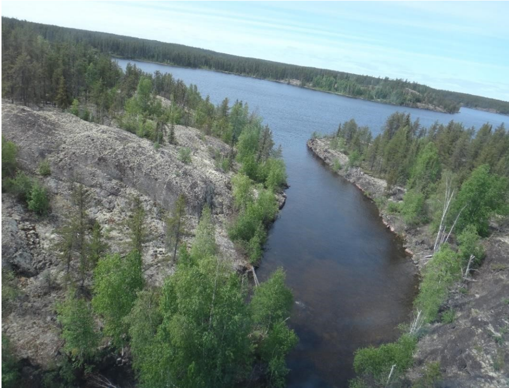
Figure D.35: Taltson Spillway 3
