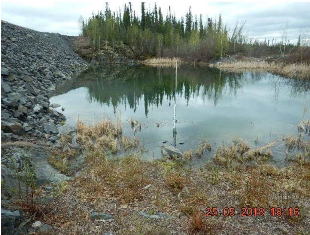
Figure D.24: Snare Forks DS of Forks Main Dam pond level monitoring gauge
