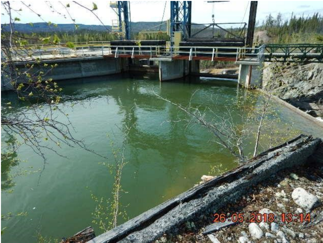
Figure D.11: Snare Falls spill gates
