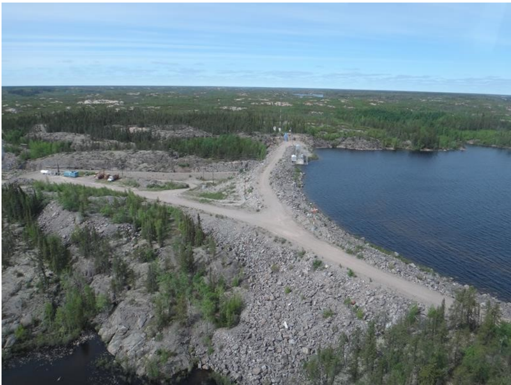
Figure D.32: Taltson Main Dam
