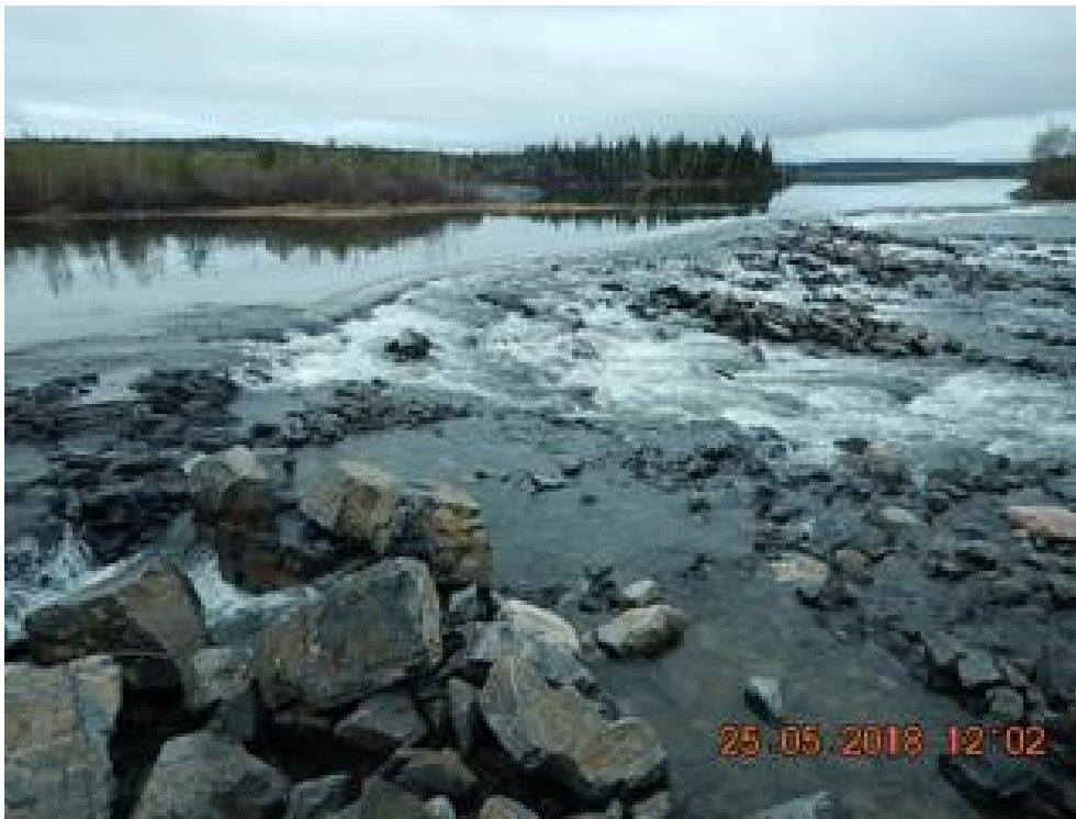
Figure D.22: Snare Forks Spillway
