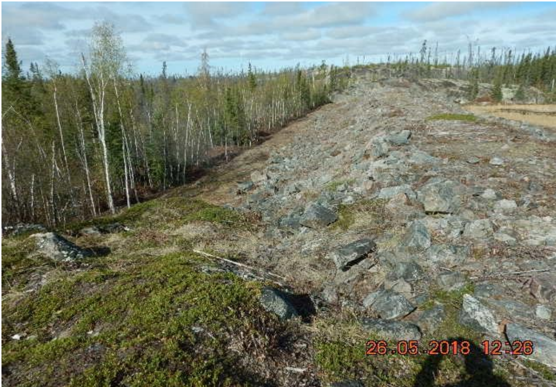
Figure D.13: Snare Falls Side Dam # 2 Downstream
