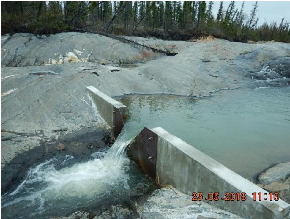
Figure D.23: Snare Forks Dyke 1 seepage weir
