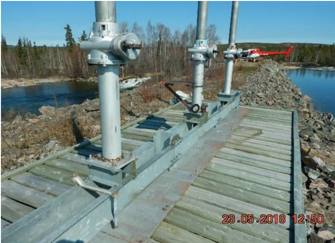
Figure D.28: Nonacho intake structure
