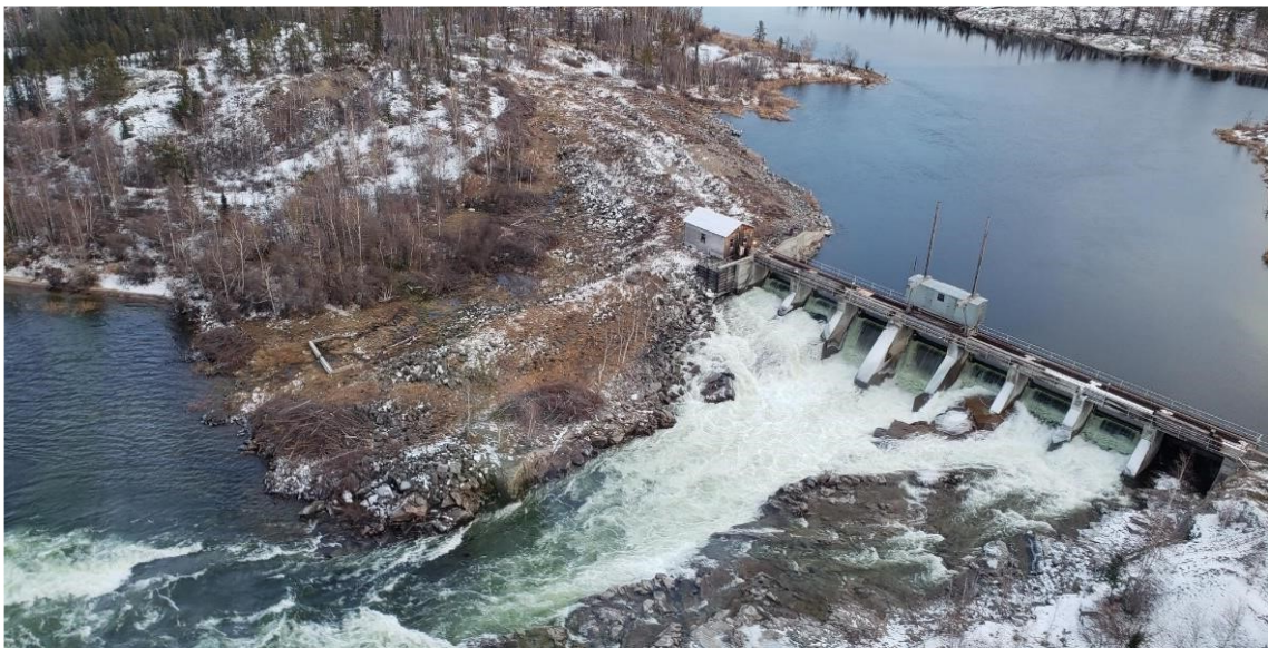
Figure D.6: Snare 5B Spillway & Dam
