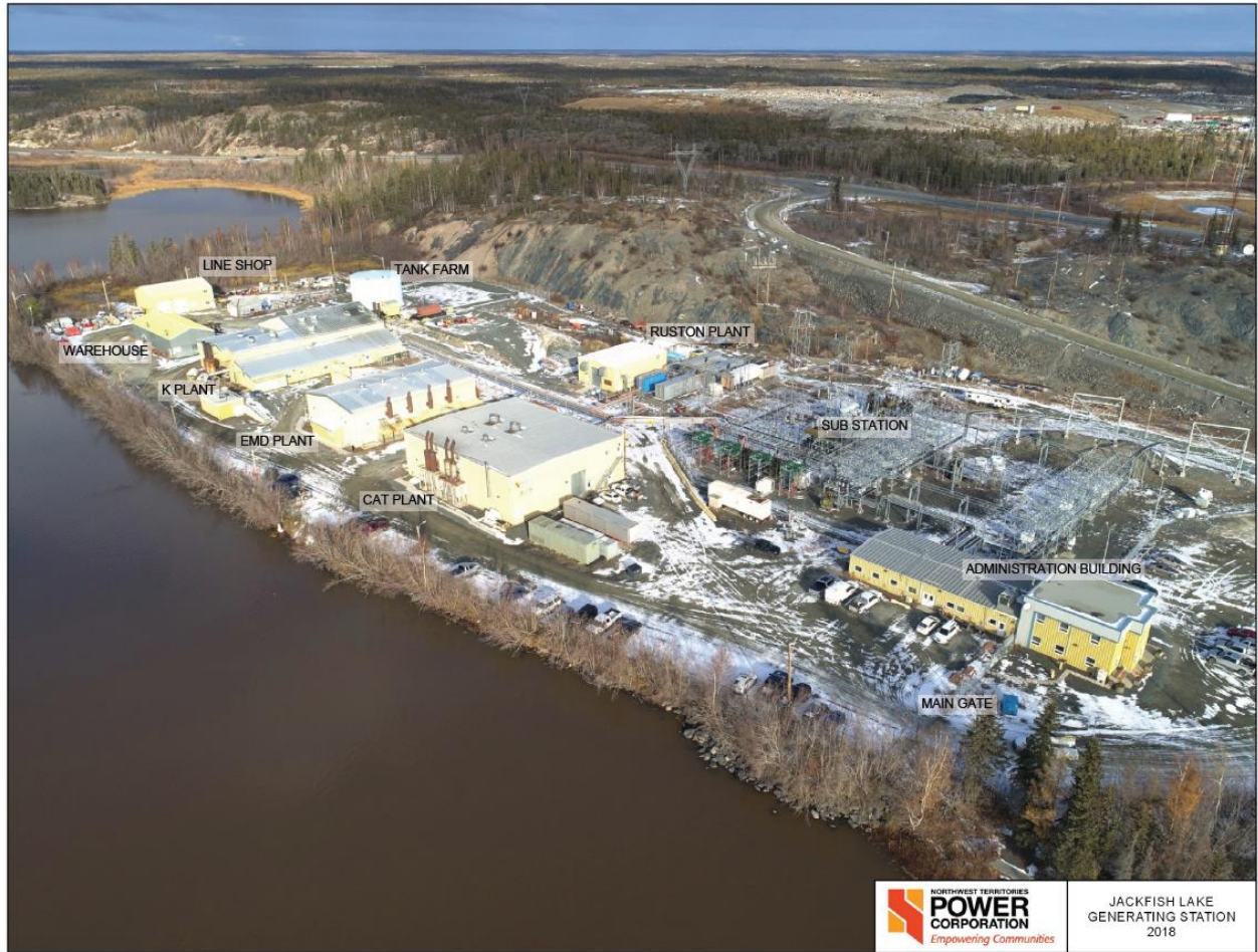
Figure 2-1: Jackfish Lake Generating Facility
