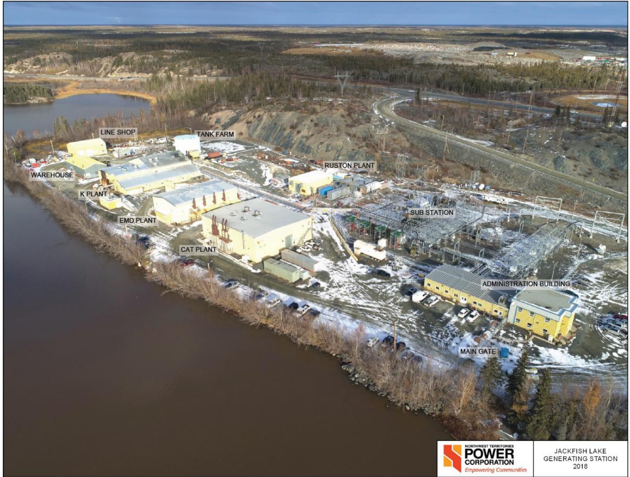
Figure 3: Jackfish Lake Generating Facility
