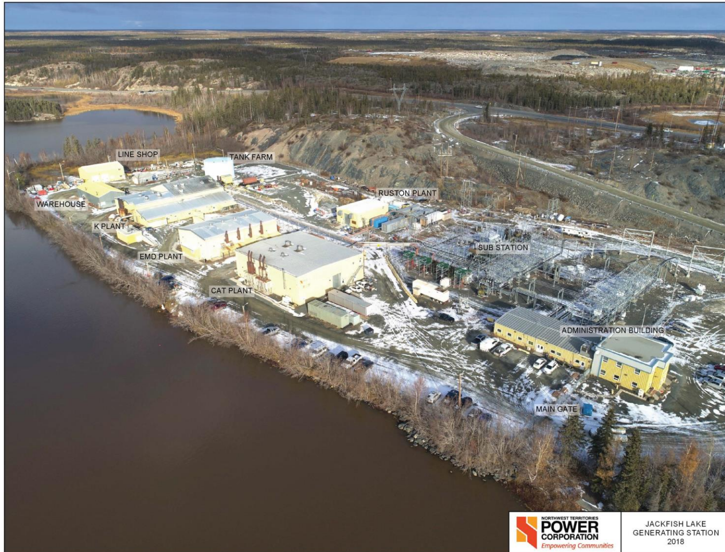
Figure 4: Jackfish Lake Generating Station Aerial
