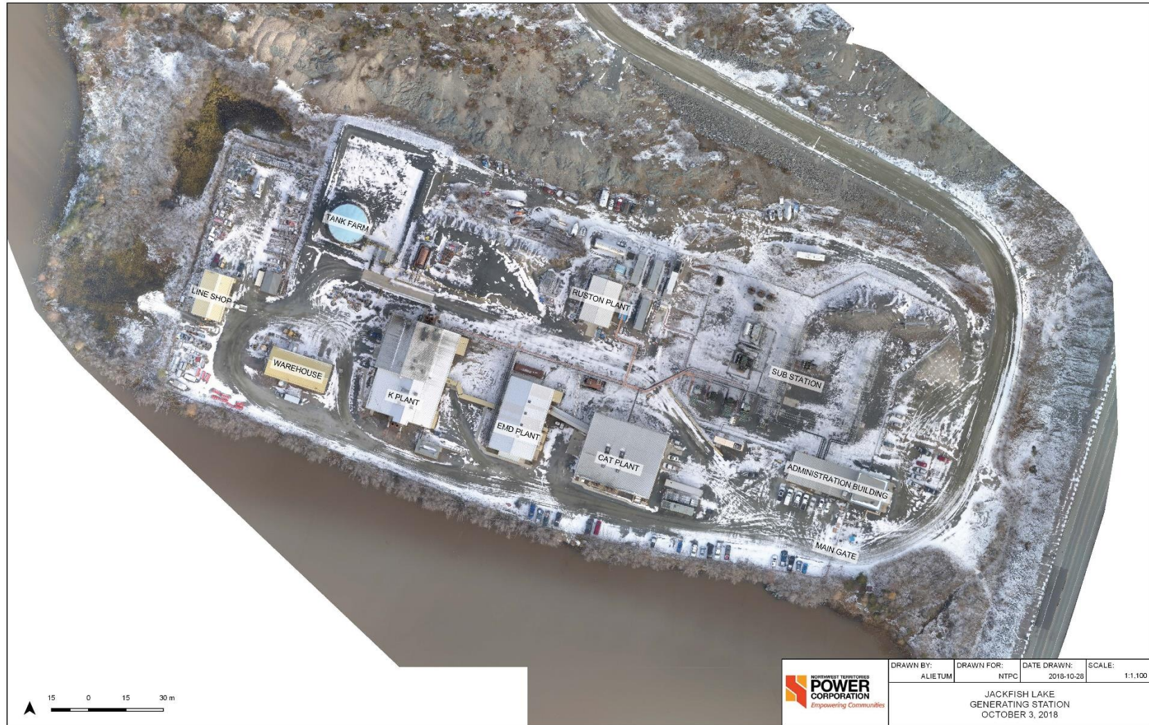
Figure 3: Jackfish Lake Generating Station Overview
