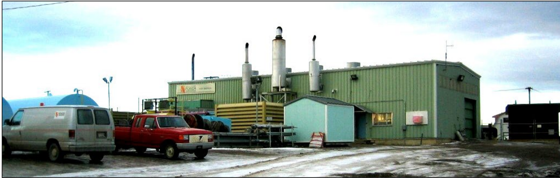
Figure 2: Fort Simpson Plant
