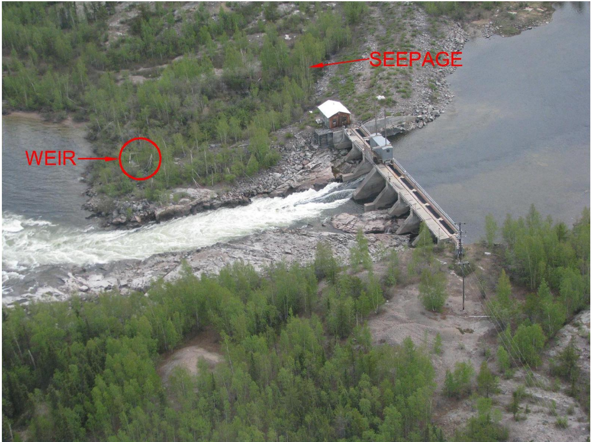
5B Spillway Seepage and Weir Location
