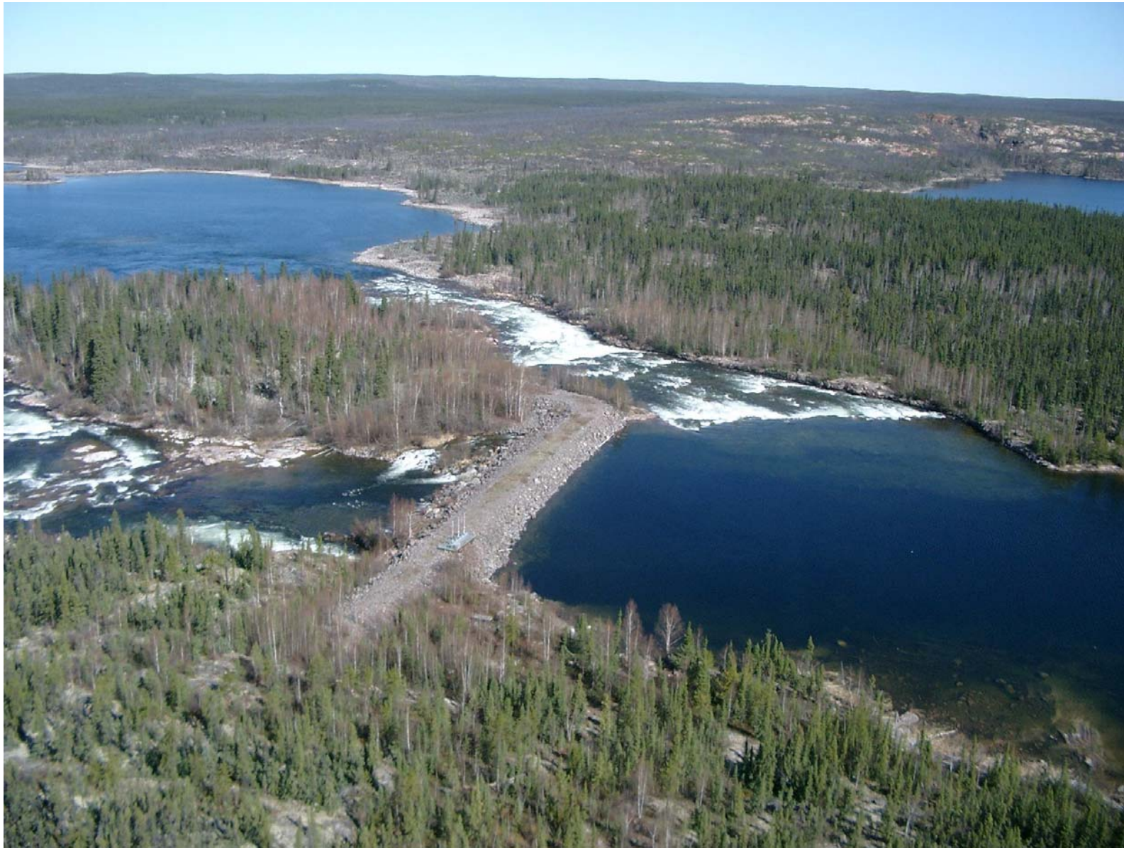
Nonacho Lake Control Structure
