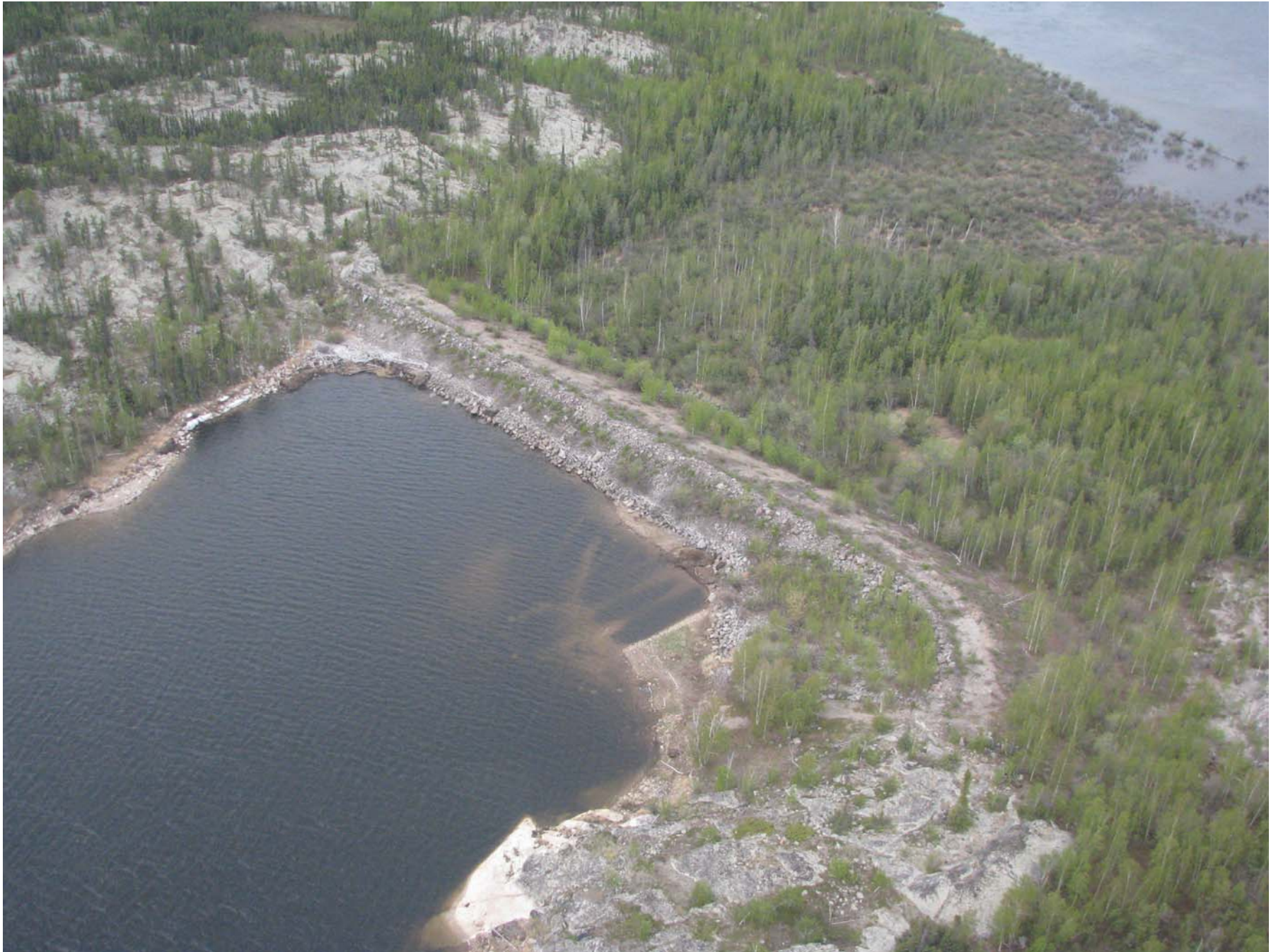
Side Dam 4 – Aerial Photo
