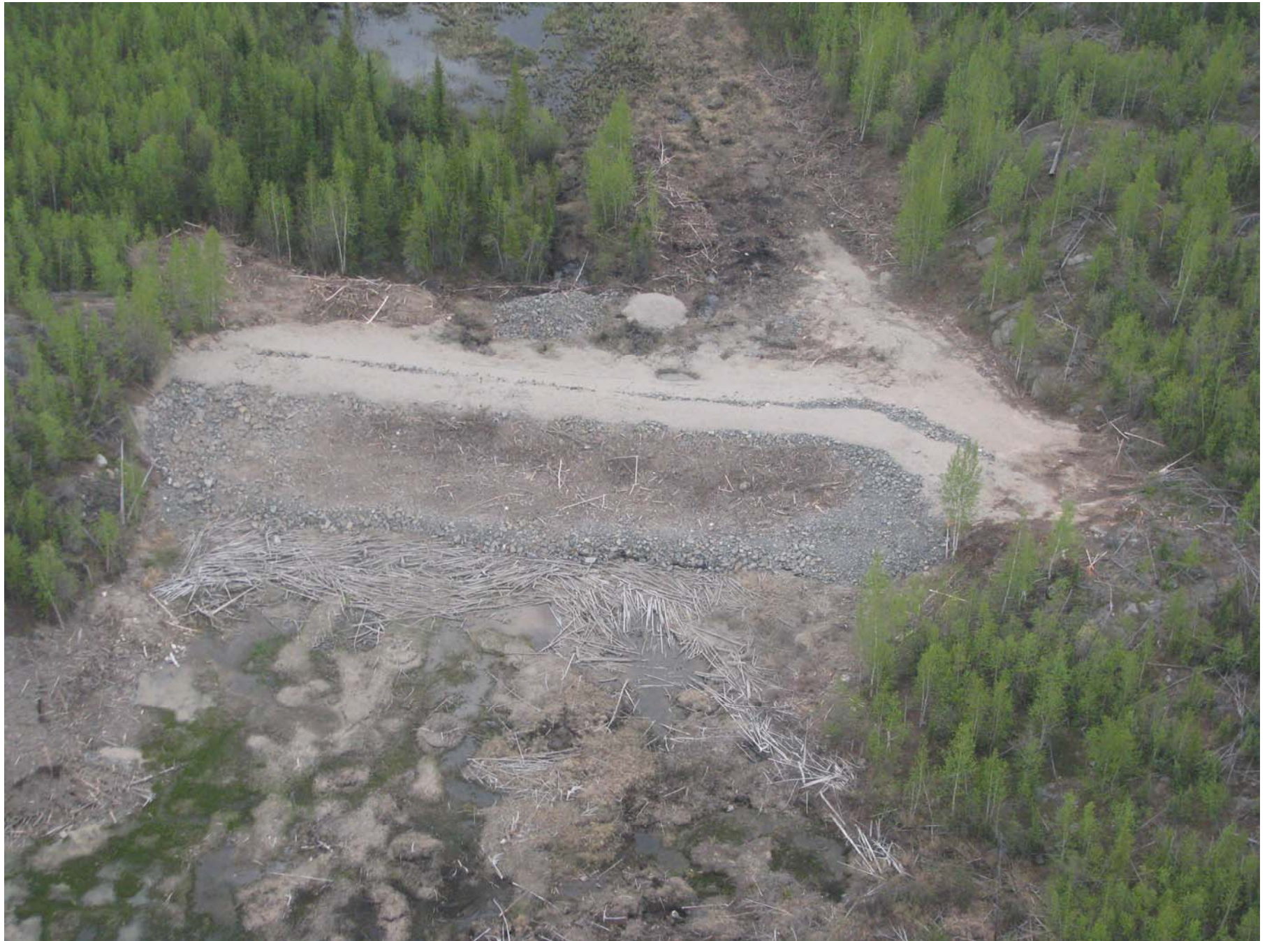
Side Dam 9B – Aerial Photo (Upstream Face Shown)
