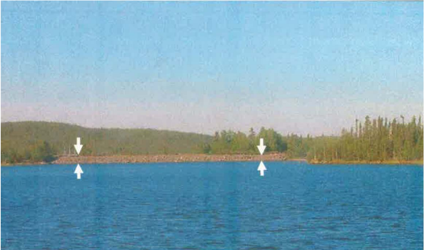
Settlement on the right near the right abutment
