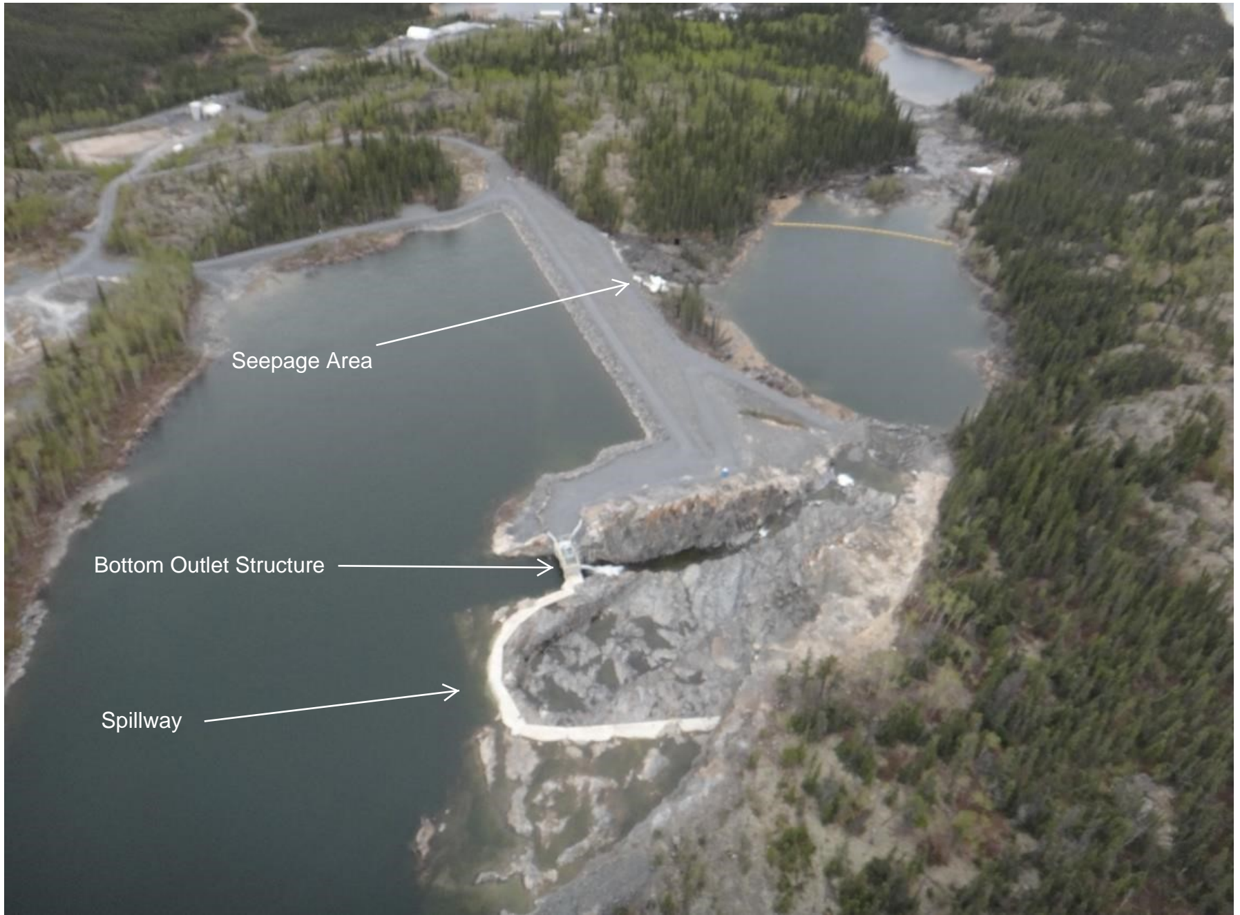
Bluefish Dam Aerial View
