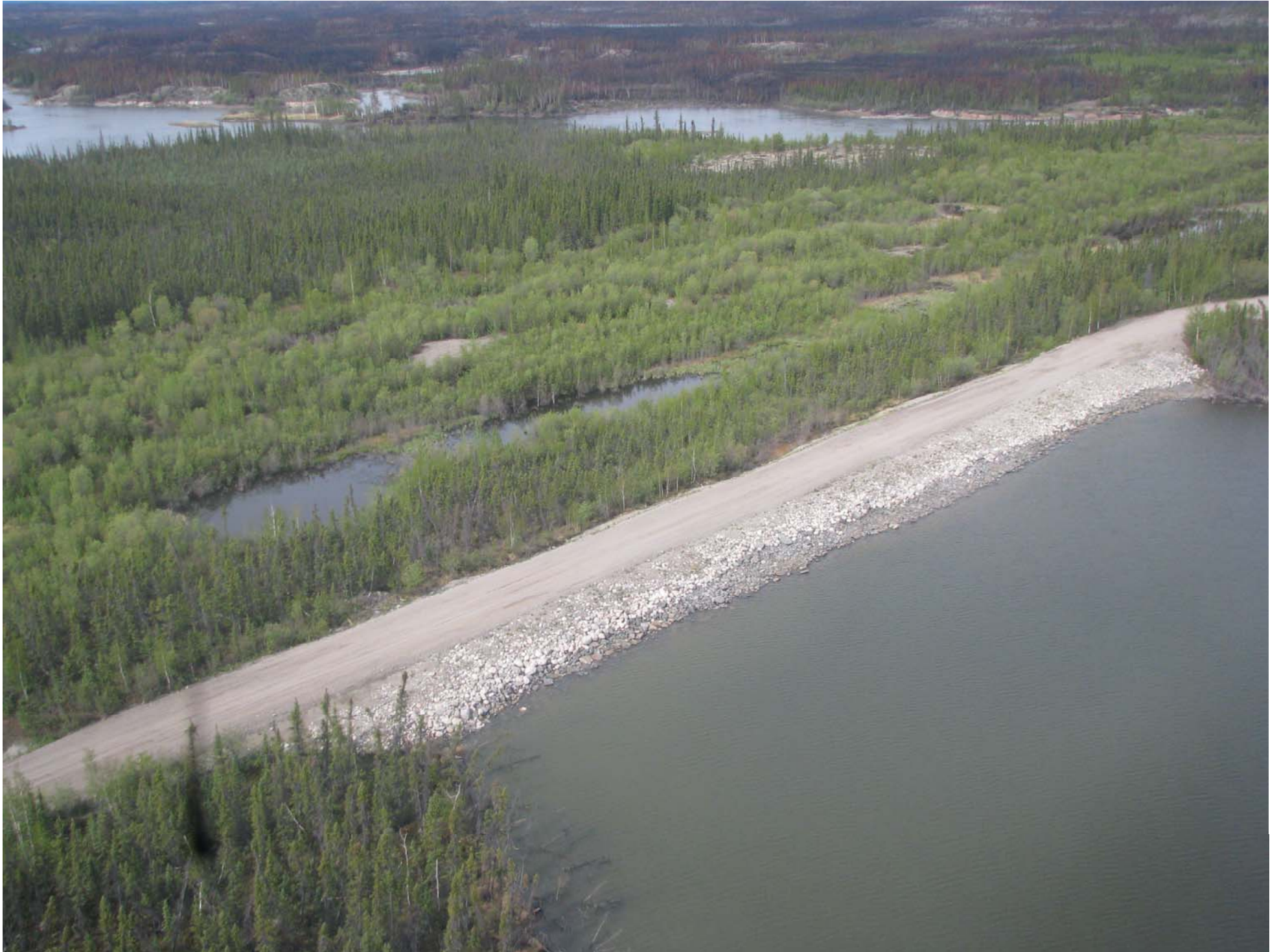
Forks Dyke #2 – Aerial Photo
