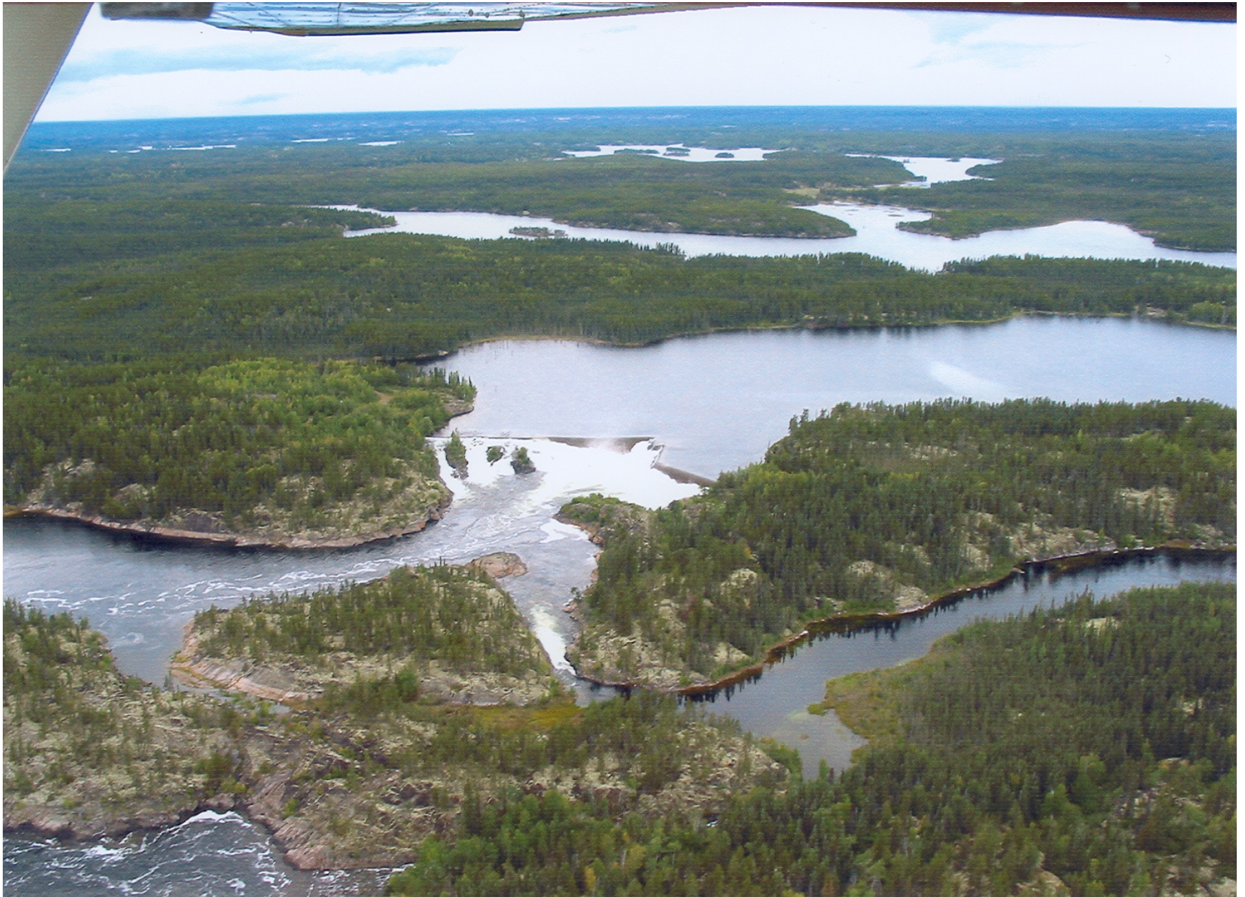
South Valley Spillway – Aerial Photo
