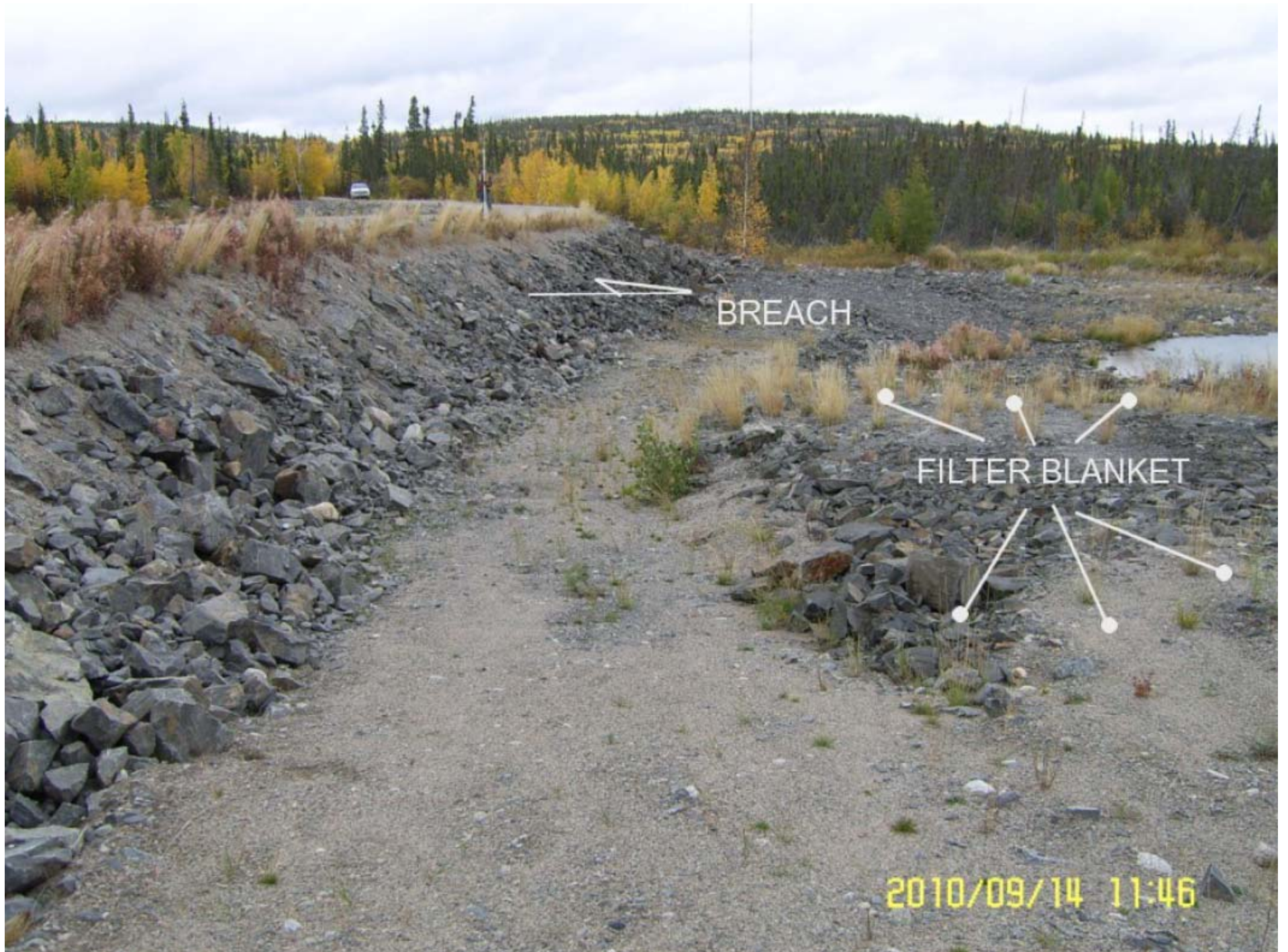
Snare Forks Dyke #1 – Seepage & Filter Blanket Location
