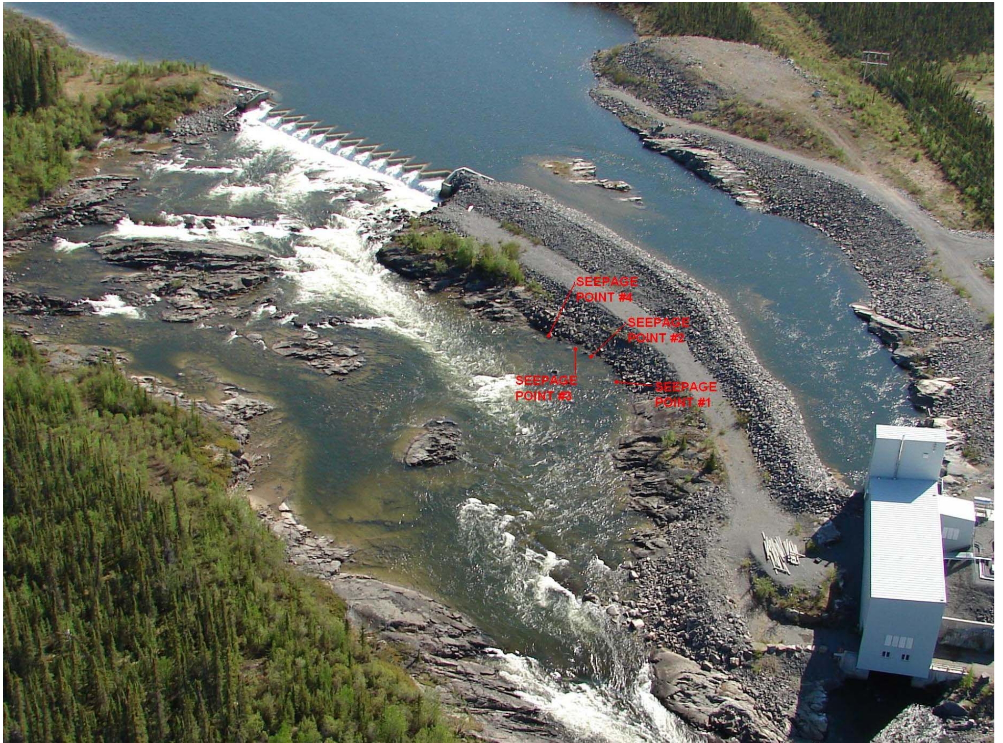
Snare Cascades – Seepage Locations
