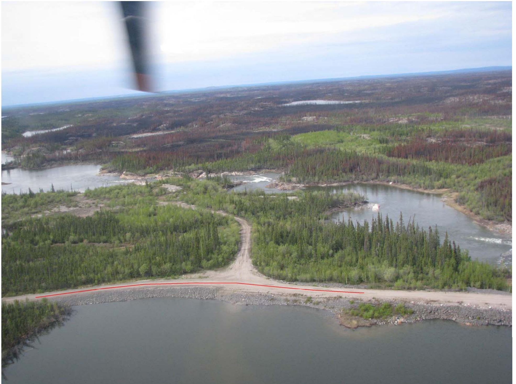
Forks Dyke #3 – Aerial Photo
