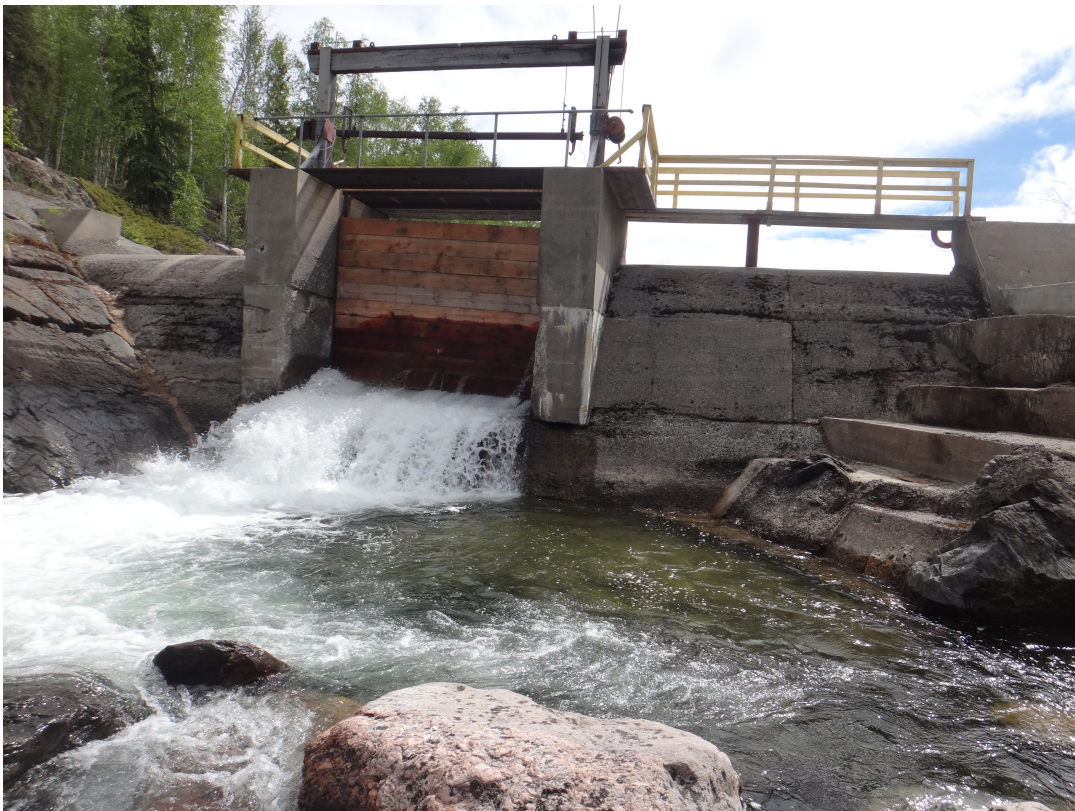
Duncan Dam Downstream
