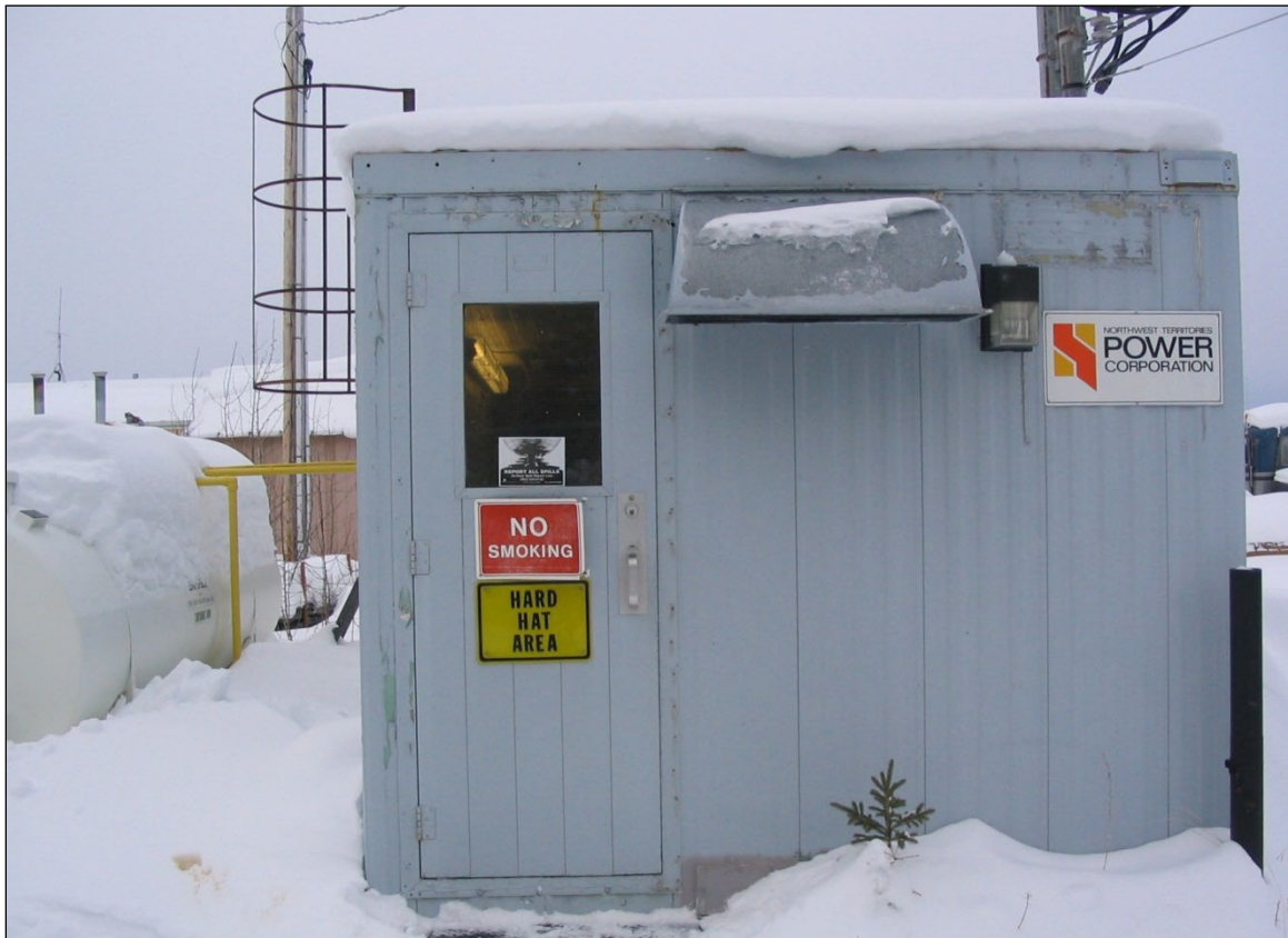
Figure 2: Buffalo Junction Plant
