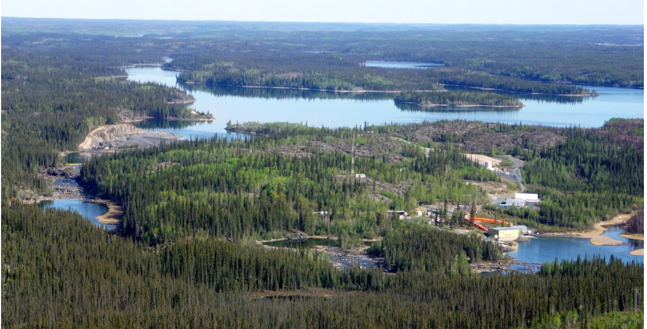
Figure 6: Bluefish Hydroelectric Facility
