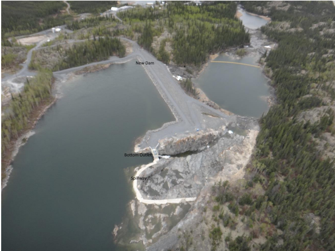
Figure 8: Bluefish Dam and Spillway
