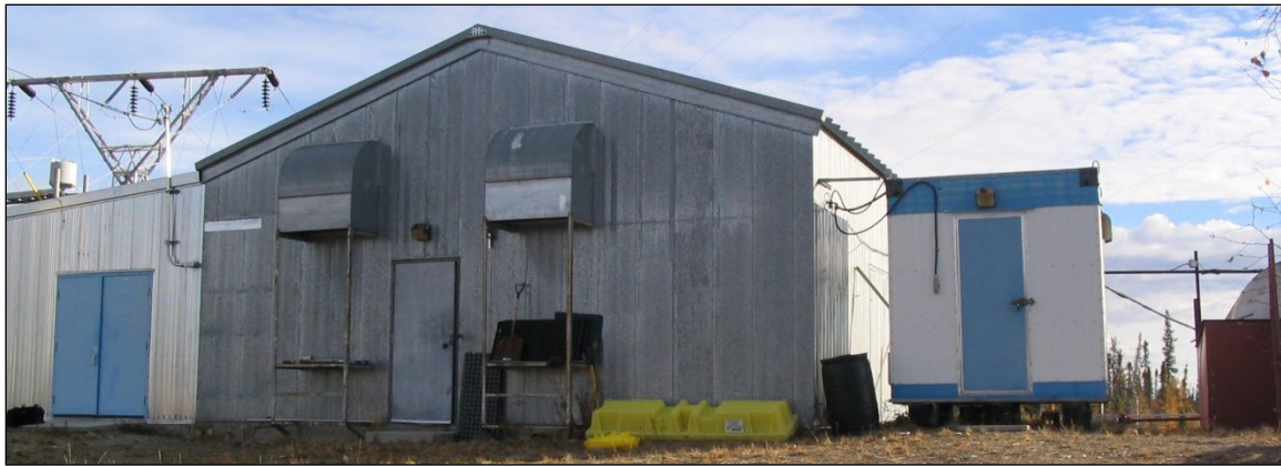
Figure 2: Franks Channel Standby Plant
