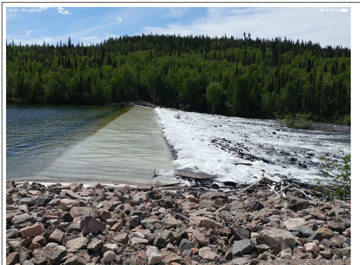
Tazin Lake Overflow Weir (From Google search) (NWT Power Corp, 2021)
