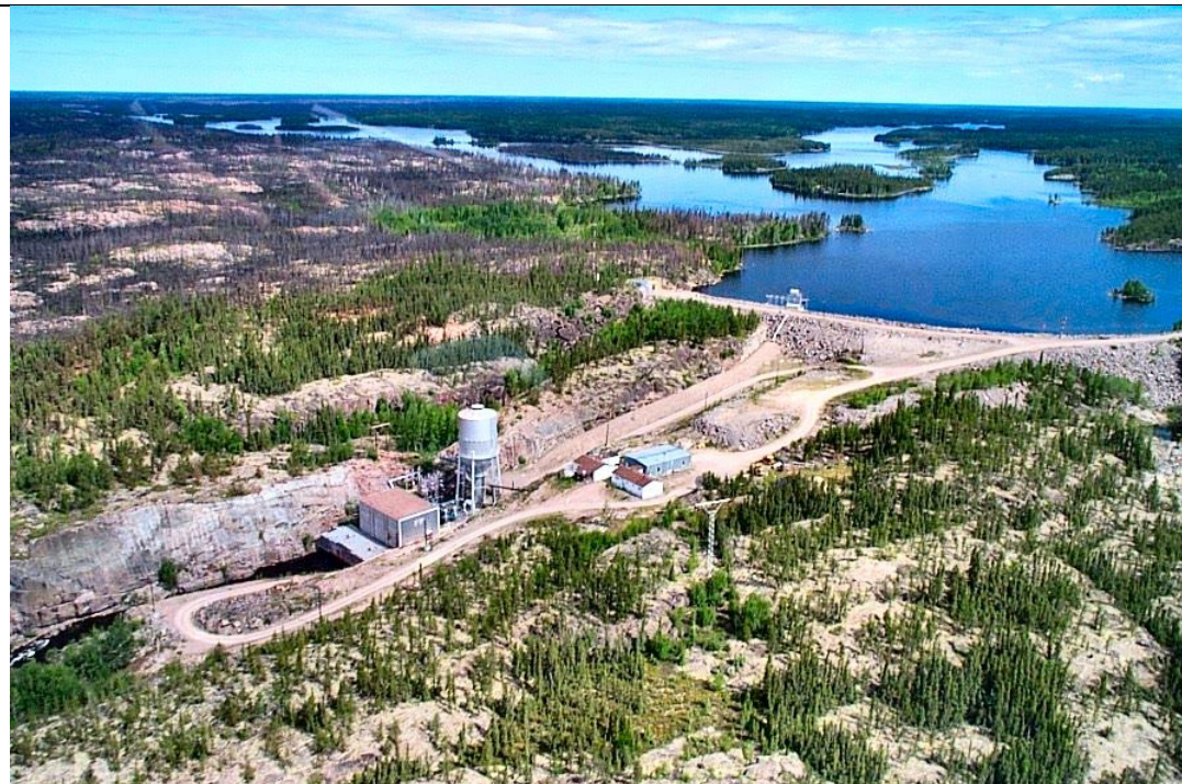
Taltson Hydro Plant (NWT Power Corp, 2016)
