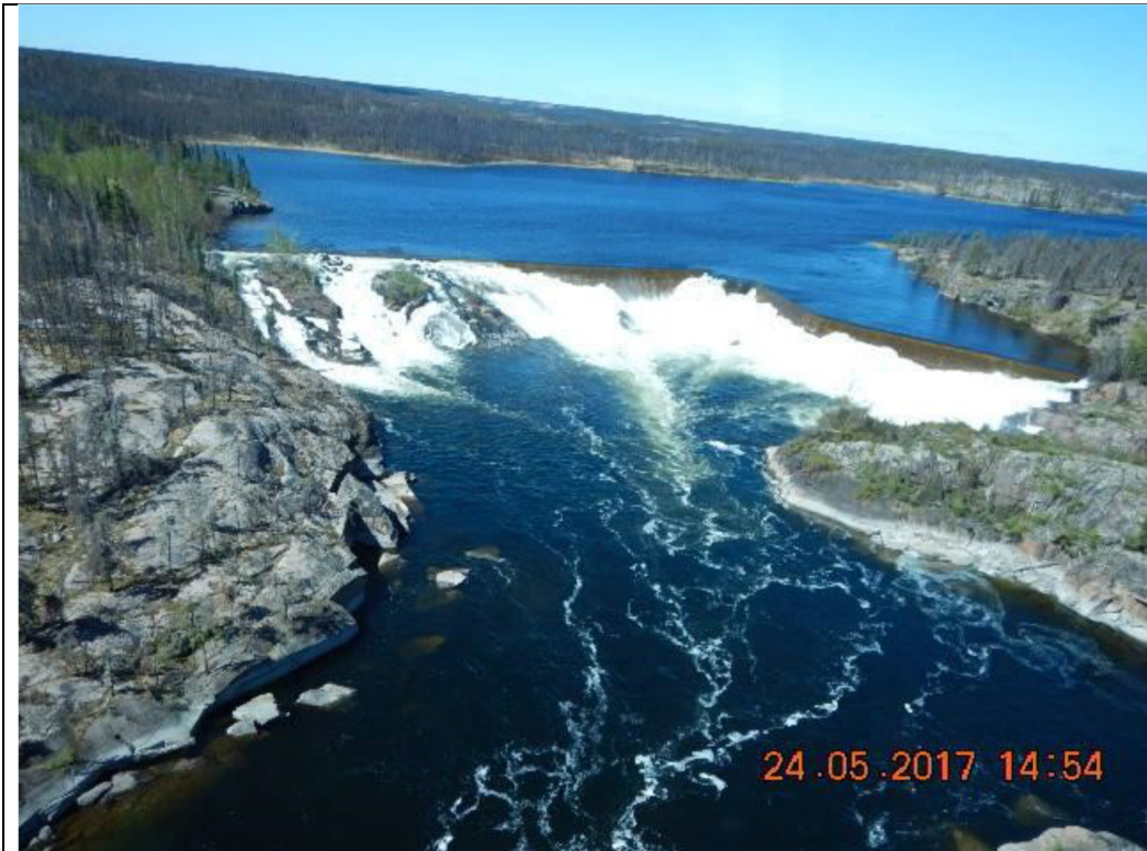
Taltson Main (South Valley) Spillway
